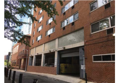
Looking NE - River West Parking Garage
