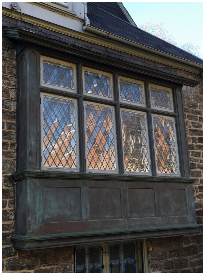
Detail of 4501 Spruce Street (façade along 45 th Street) of a cantilevered window clad in copper and diamond-pane windows.
