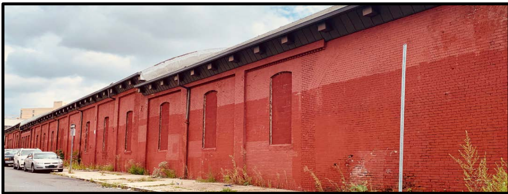
Figure 10. The west elevation of Buildings 2 and 5. Source: Oscar Beisert, 2019.
