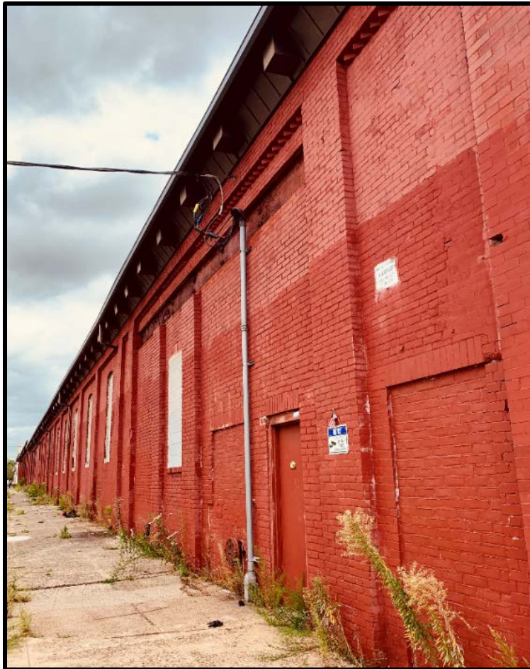
Figure 15. Top: The west elevation of Building 5. Source: Pictometry, Atlas, City of Philadelphia, 2019. Figure 16. Center: The entire west elevation of Building 5. Figure 17. Bottom: Looking north along the west elevation of Buildings 2 and 5. Source: Oscar Beisert, 2019.
