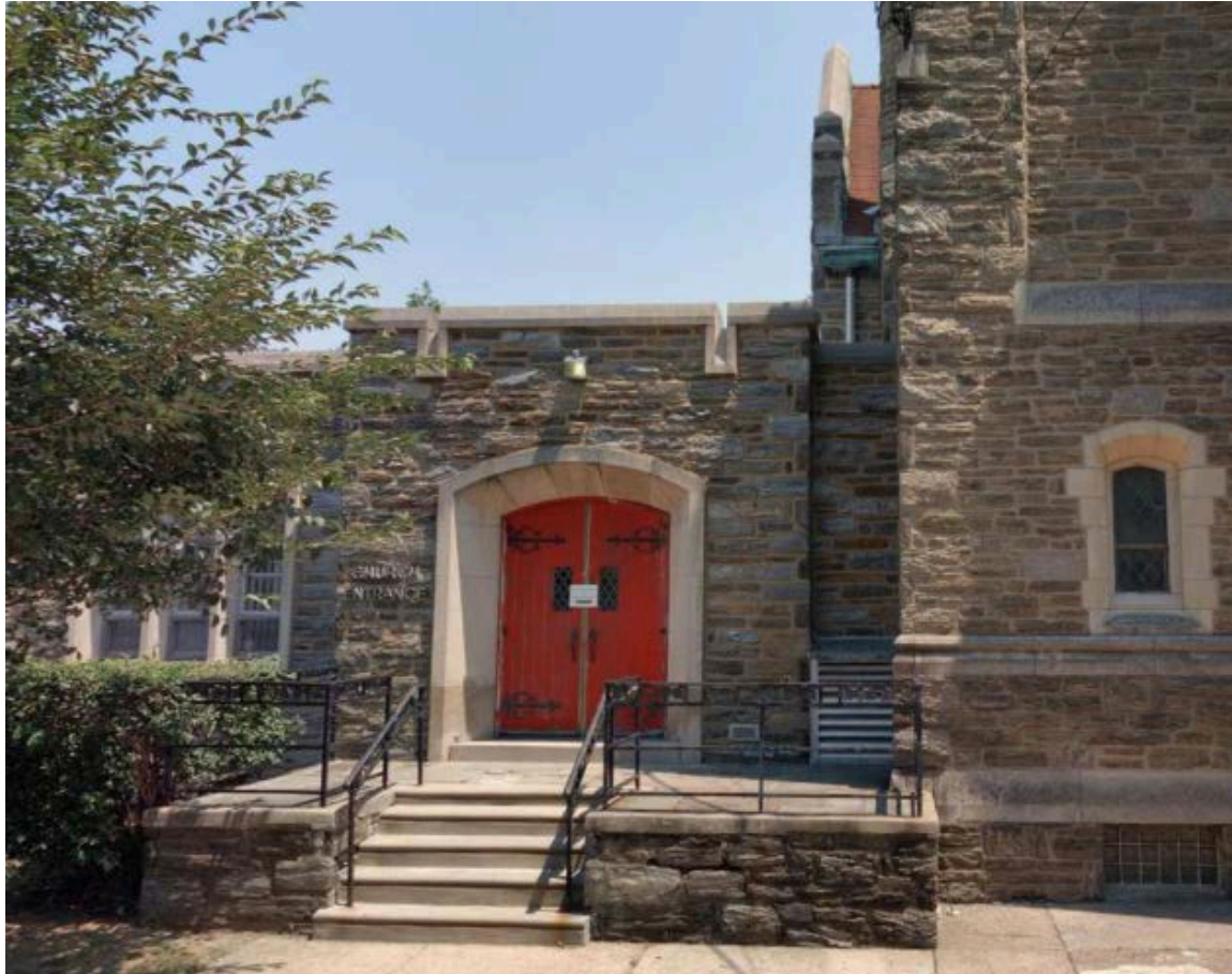
Figure 9: Detail of the connection between the addition (left) and the church. The addition is set back slightly from the plane of the church. Source: Cyclomedia, 2019.
