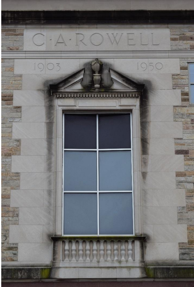
Figure 5. One of two large, two-story windows with classical details.
