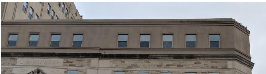
Figure 6. The fourth floor of the building, clad in dressed limestone ashlar.
