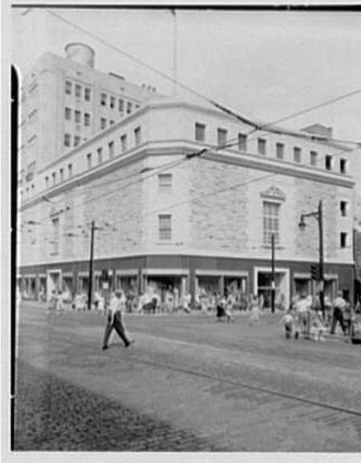
Figure 22. The Rowell Department Store as it appeared in 1950. The building's windowless massing is typical of department stores of the era.
