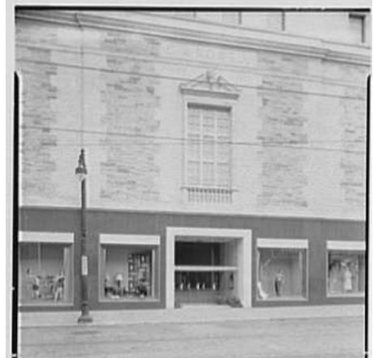
Figure 23. The Rowell Department Store's Modern first floor in 1950.
