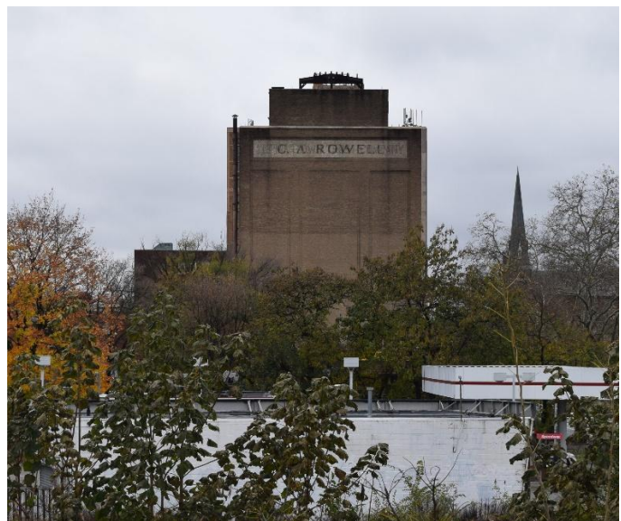
Figure 10. The rear elevation opposite Germantown Avenue.
