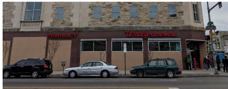
Figure 3. The first floor of the building, clad in purple-red granite and beige stucco.
