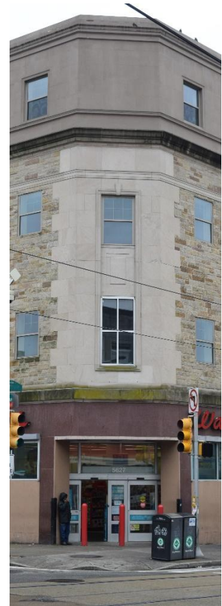
Figure 7. The canted corner of the building.
