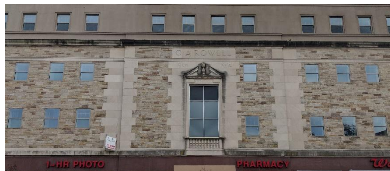
Figure 4. The second and third floors of the building. Note the quoining and quarry-faced limestone.
