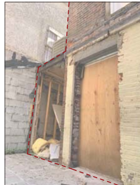
4 LOOKING AT BUILDING REAR FROM REAR ALLEY REMAINING 1-STORY ADDITION & REAR WALL TO BE DEMOLISHED
