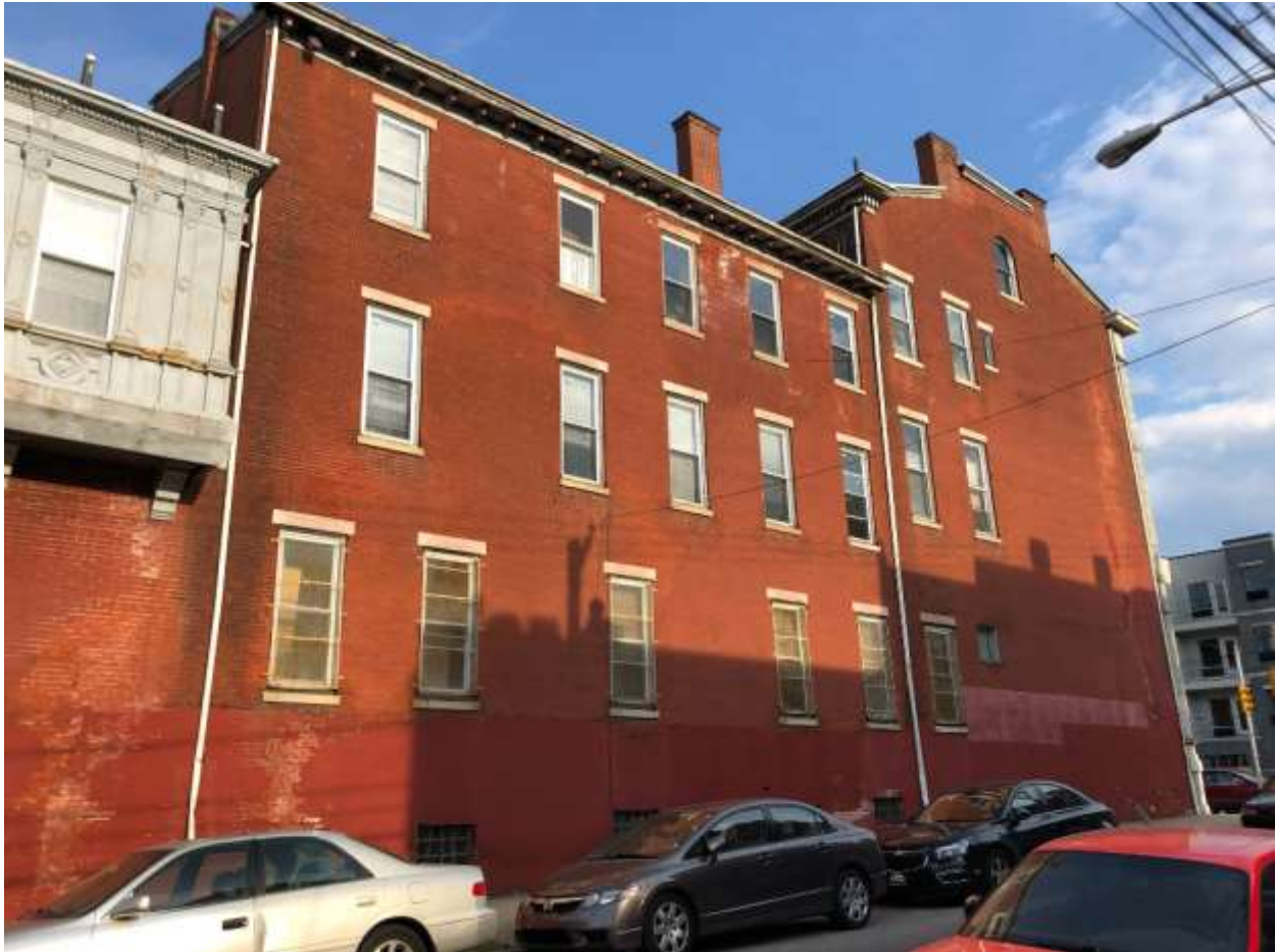
Figure 3: West elevation along 16 th Street, showing the main block (to the right), the three-story rear extension (center), and a portion of the two-story rear extension (to the left), May 2019.
