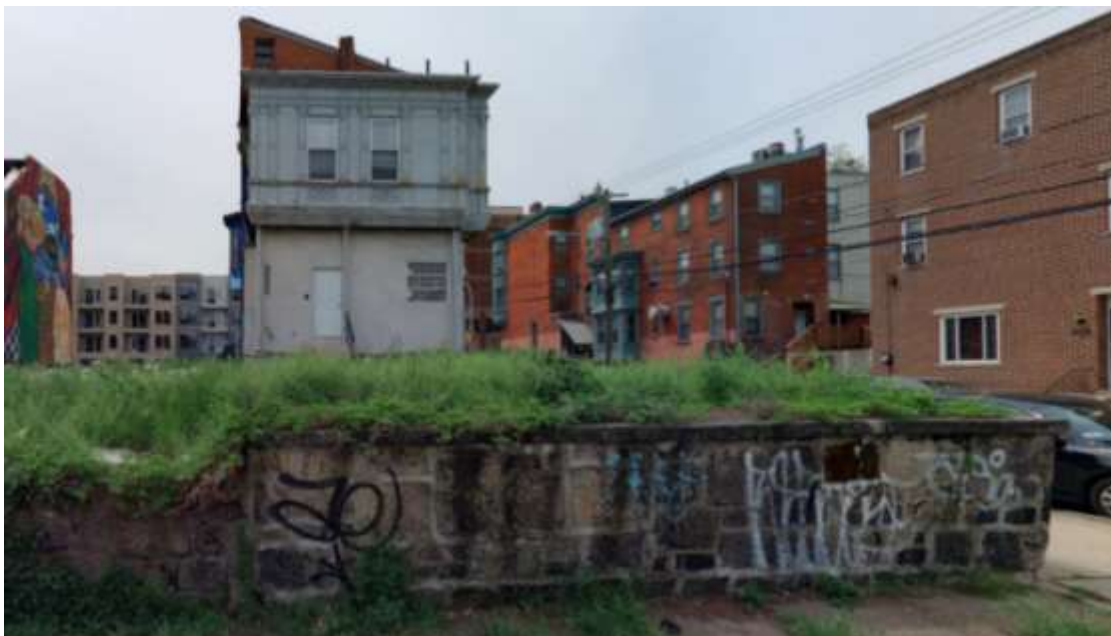
Figure 5: View south towards the rear, north elevation of the property from Flora Street, May 2019.
