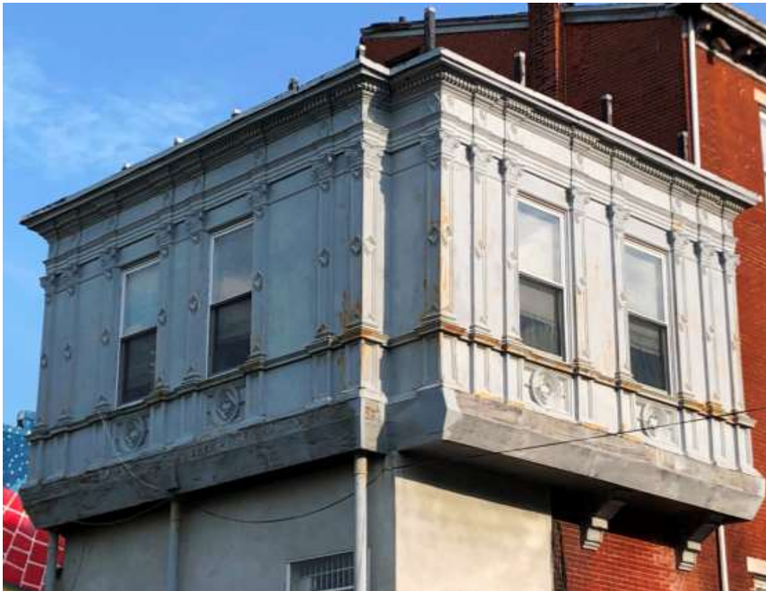
Figure 6: Details of the metal-clad second-floor rear extension, May 2019.
