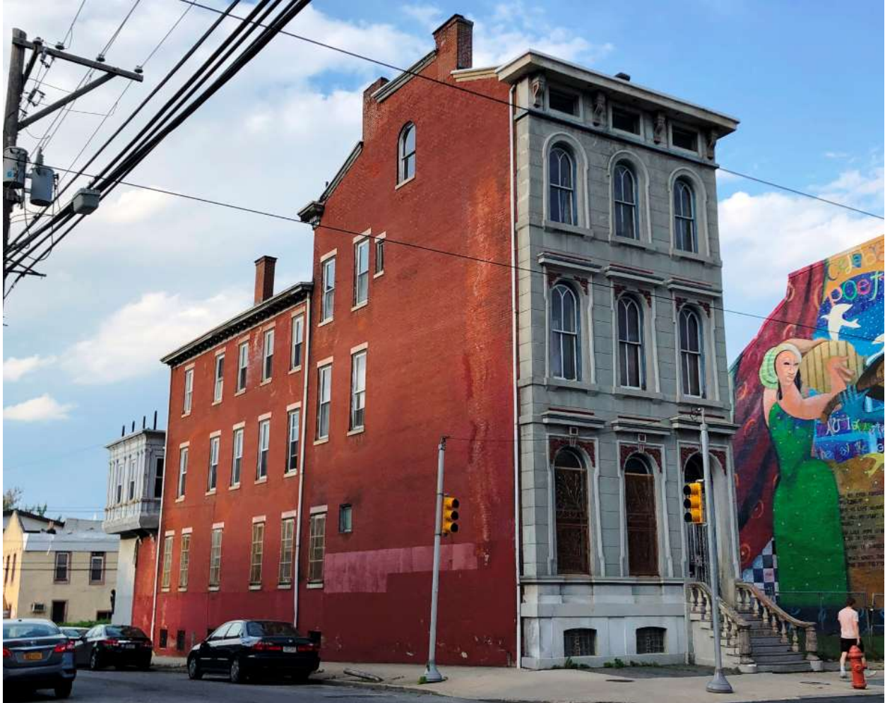
Figure 1: View of 1535 W Girard Avenue looking northeast from the intersection of Girard Avenue and N 16 th Street, May 2019.
