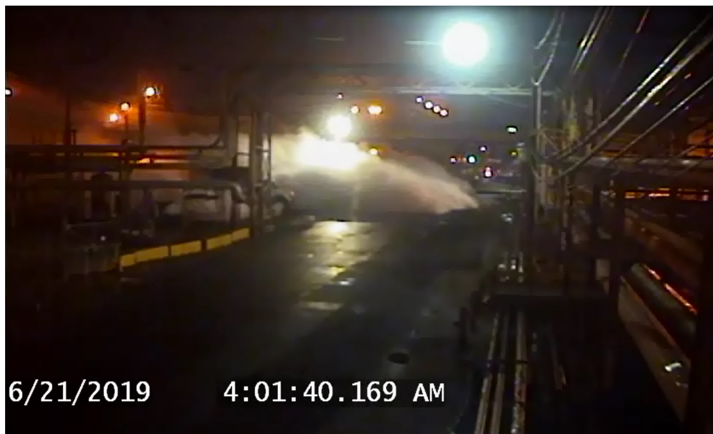
Figure 3. Security camera footage of leaking process fluid. It formed a large ground-hugging vapor cloud that surrounded some sections of the unit. (Credit: PES).
