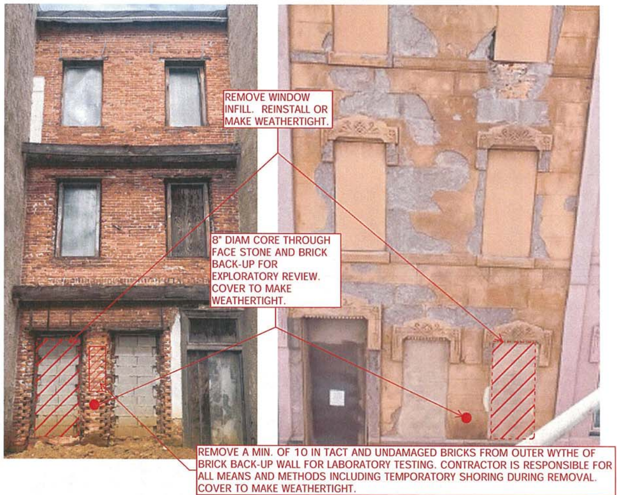
Figure 1: Photographs of the front and back of the building showing the location from which the samples were taken, and condition of the bricks in the field.
