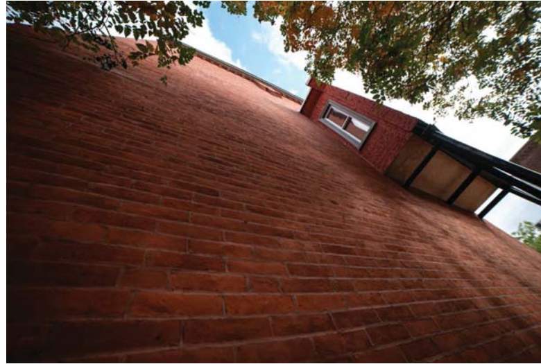
Side facade on the alley
