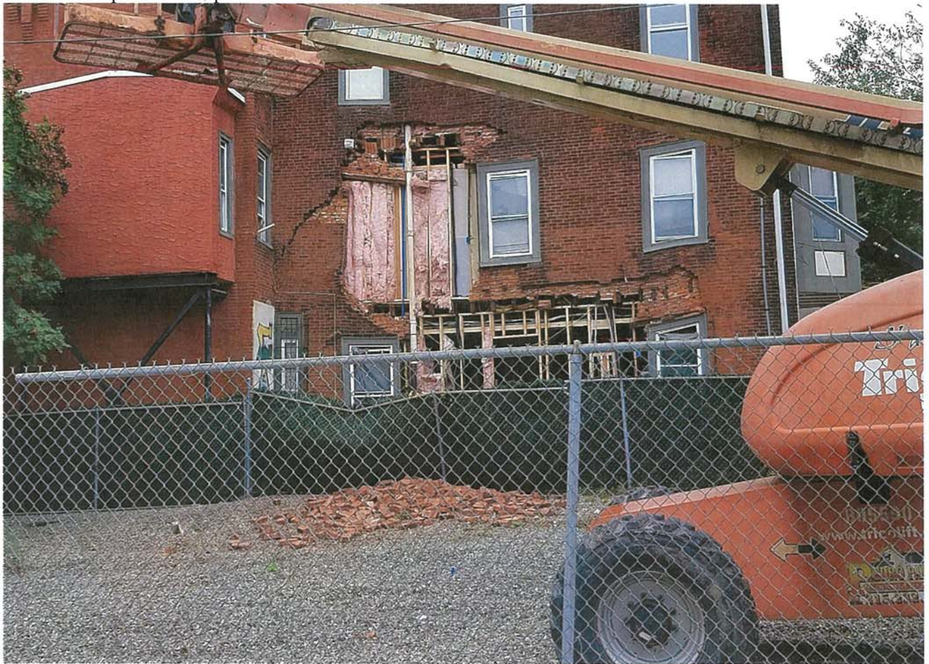
Partial collapse of wall; prior to demolition
