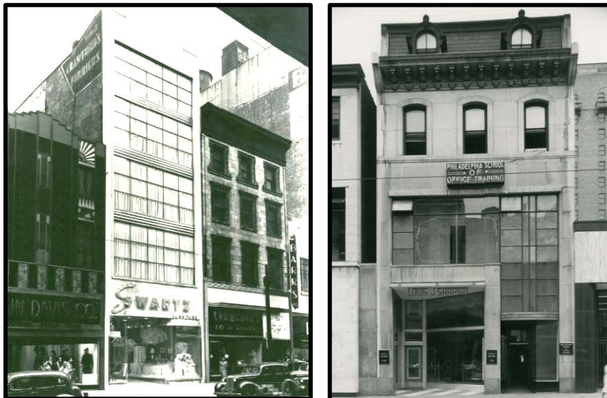
Figure 17. Left: The Davis Company at 704 Chestnut street (to the far left in the photograph) featured a façade of glass panels, which was somewhat unusual in that it covered a three-and-one-half-story elevation—basically rising to the full height of an existing townhouse (c1800). While this façade was listed on the Philadelphia Register of Historic Places, it was destroyed c2013. Figure 18. Right: Louis J. Shapian Furs, featuring a storefront alteration at the first and second floors, exhibiting the results of modernizing older residential buildings with the open front without standardized designs and motifs. The date of this alteration is unknown to the author at this time, but the photograph was taken in 1949.
