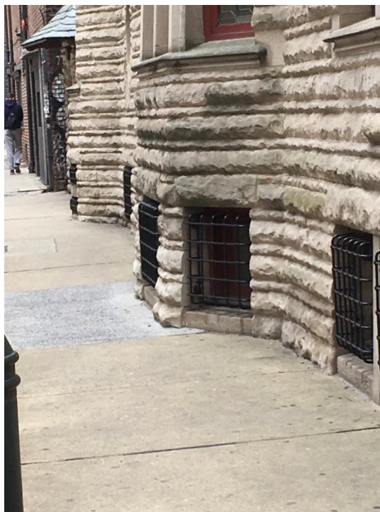
Details of the Moore House showing Eyre's use of stone and brick, stone detailing, wall projections, iron grilles, stone lintels, and diamond-shaped panes. Notice the plastic qualities of the stone wall.
