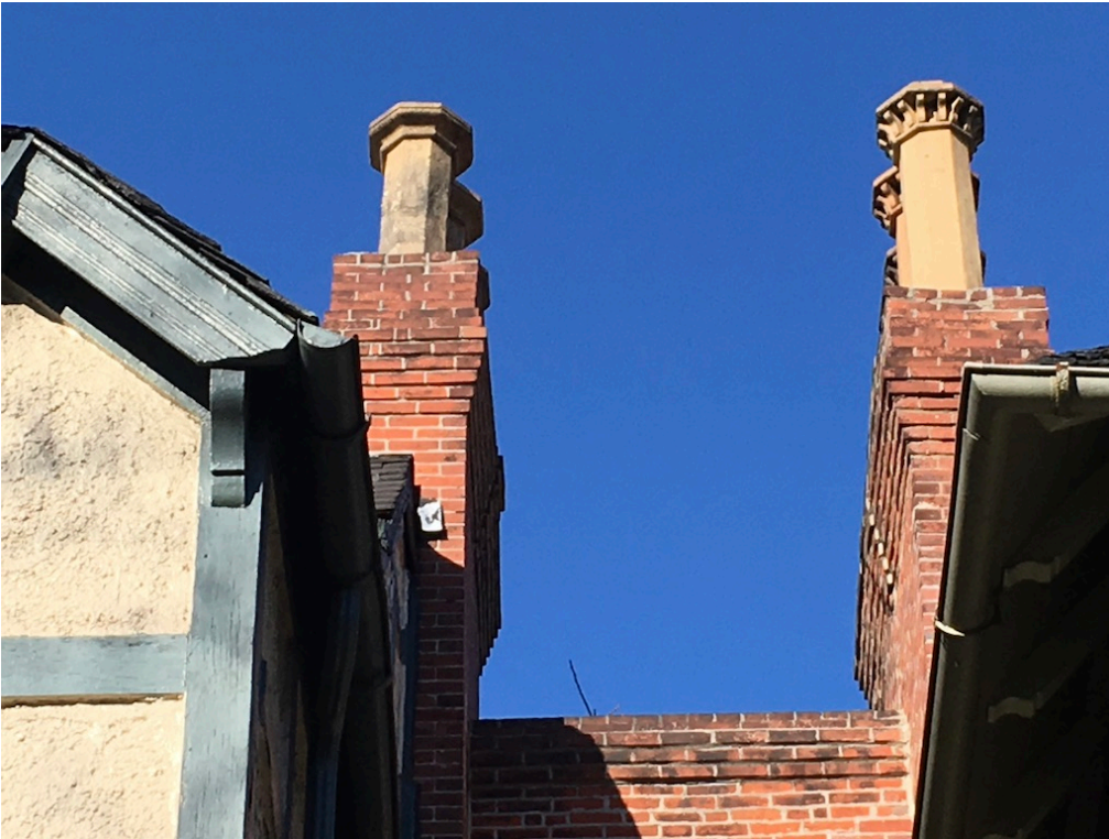
Detail of 4505 and 4507 Spruce Street of corbelled, decorative chimneys with the archway connecting them.
