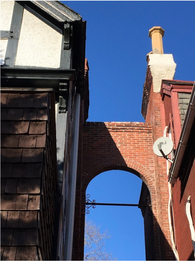
Detail of 4505-4507 Spruce Street with a corbelled chimney and chimney pot, brick arch connector, steep slate roof (on right), and cantilevered third floor (on left).
