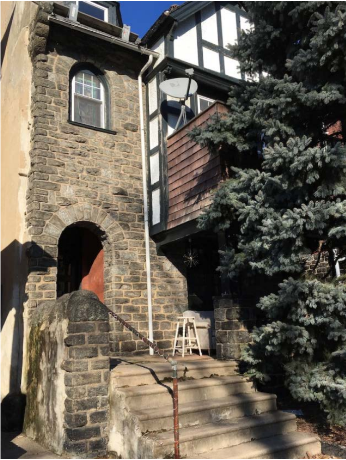
Detail of 4507 Spruce Street with stone façade, arched door and window, decorative half-timbering with stucco infill, and stone corbel and post.
