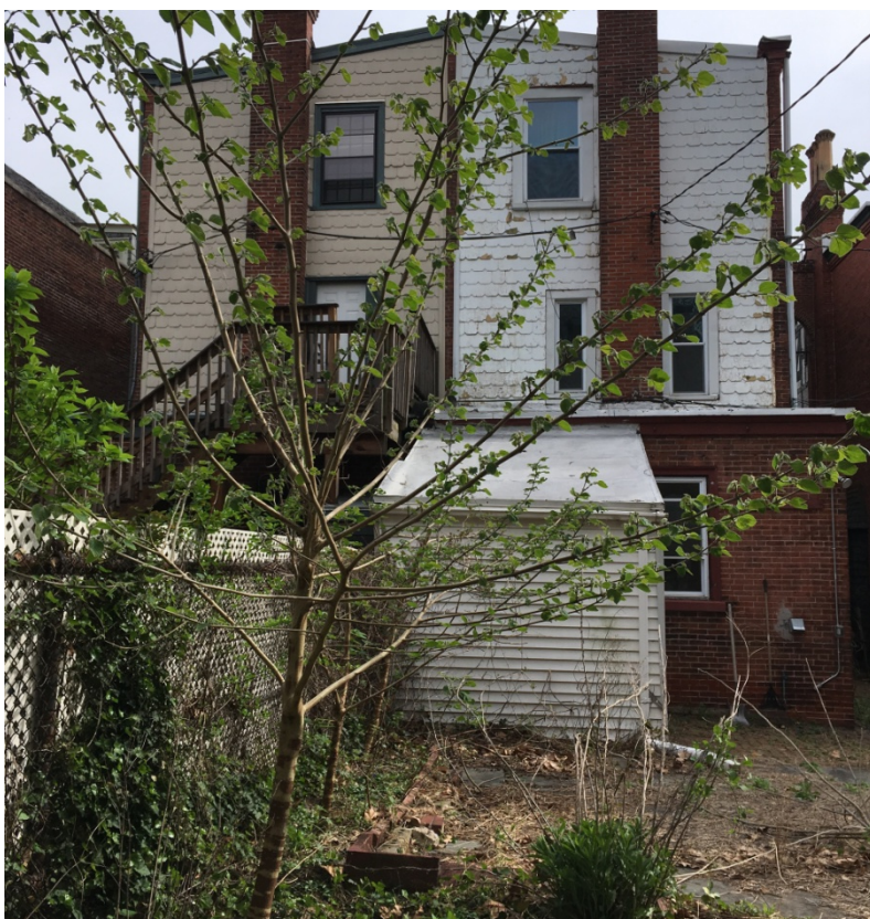
The rear view of 4503-4505 Spruce Street showing the nearly sloped roof and the first floor laundry room in brick. The white clapboard ell is a later addition. The first floor laundry can also be seen on the left – belonging to 4503 – under a recent roof deck and stair renovation.
