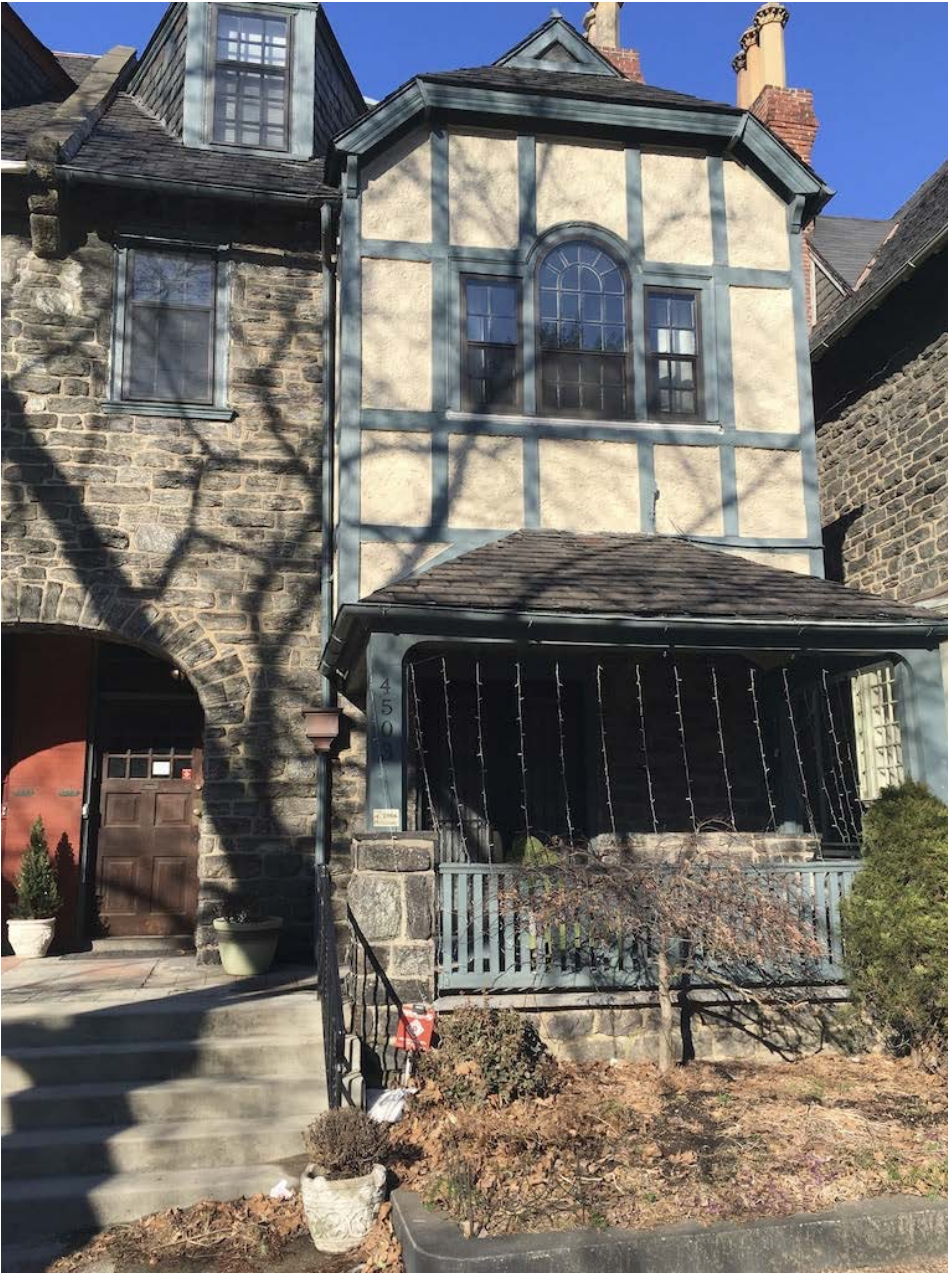
4503-4505 Spruce Street showing the Palladian window divided by half-timbering.
