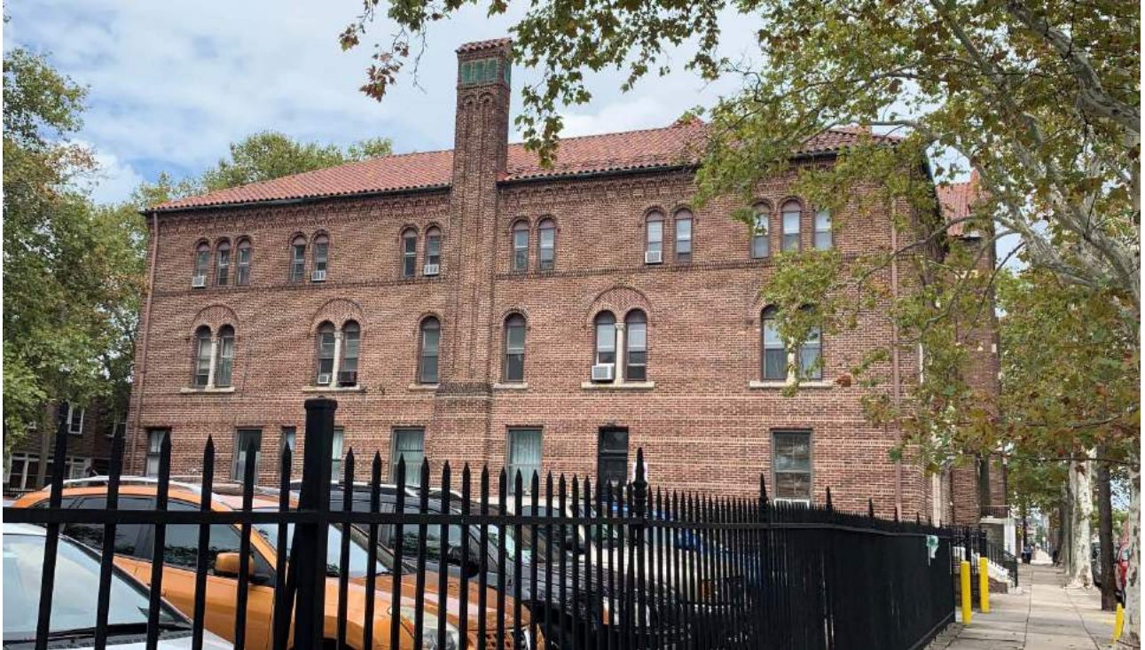
Side (south) elevation of rectory from S. 21 st Street, September 2019.
