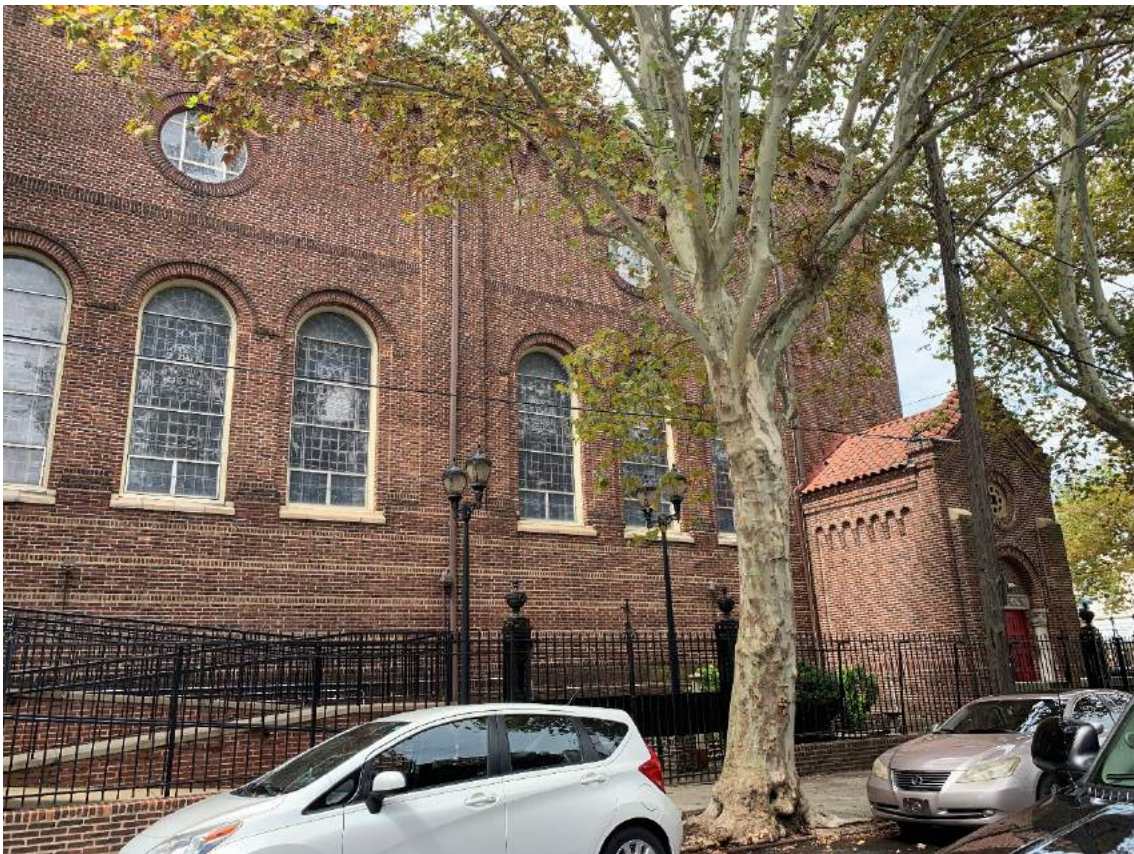
Side (east) elevation of church from S. 21 st Street, September 2019.
