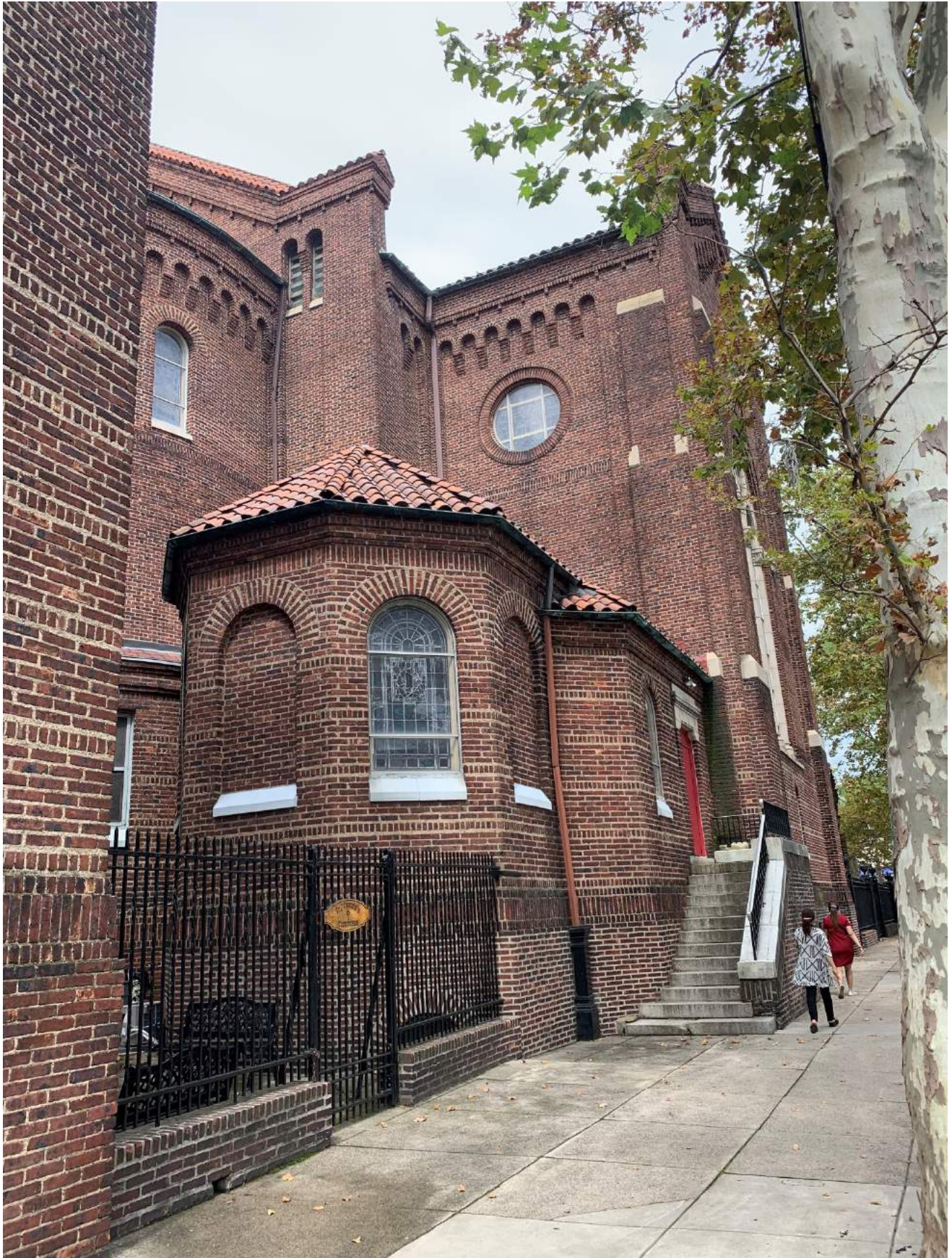
Rear (south) and side (east) elevations on S. 21 st Street, September 2019.
