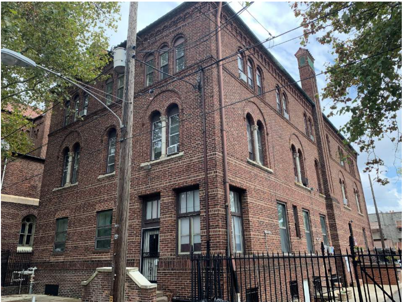
Rear (west) elevation of rectory from Norwood Street, September 2019.
