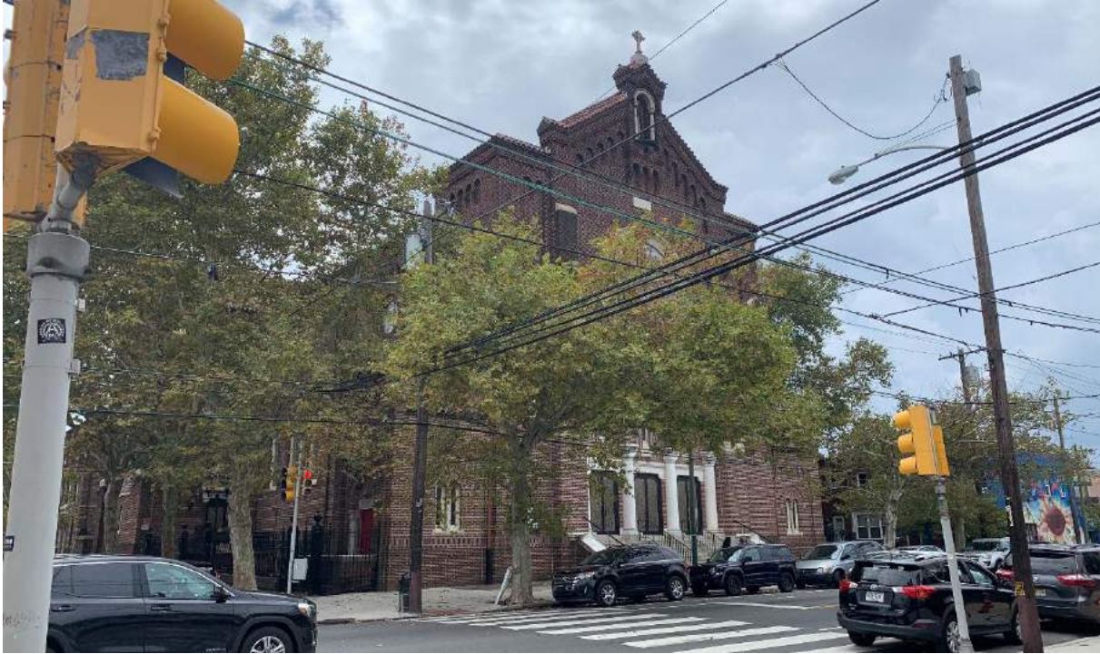
Primary (north) façade from S. 21 st Street and Snyder Avenue, September 2019.
