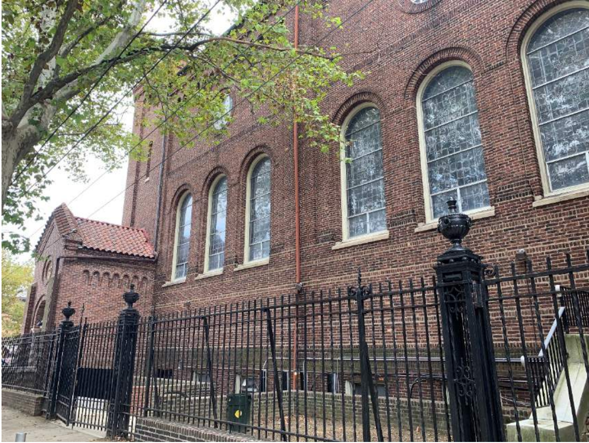
West elevation of church on Norwood Street, September 2019.
