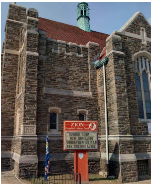
Figure 5: South elevation details, including the crenelated parapet, buttress detailing, and cornerstone (left), and the entrance bay details (right). Source: Cyclomedia, July 2019.
