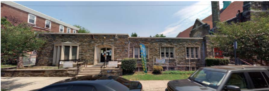
Figure 10: The west elevation of the addition is six bays wide and pays homage to the historic church building in materials and detailing such as the crenelated parapet, and yet is decidedly modern and of its time. Source: Cyclomedia, 2019.
