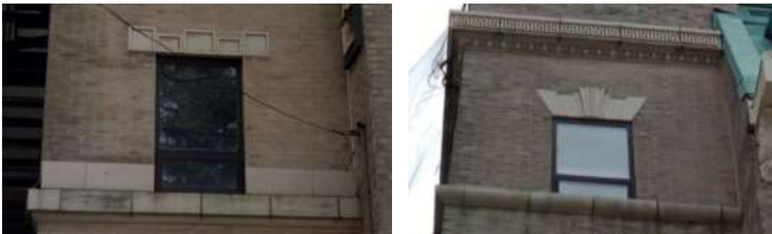
Figure 14: Details of the second and fourth-floor window openings, beltcourses, and terra cotta detailing.
