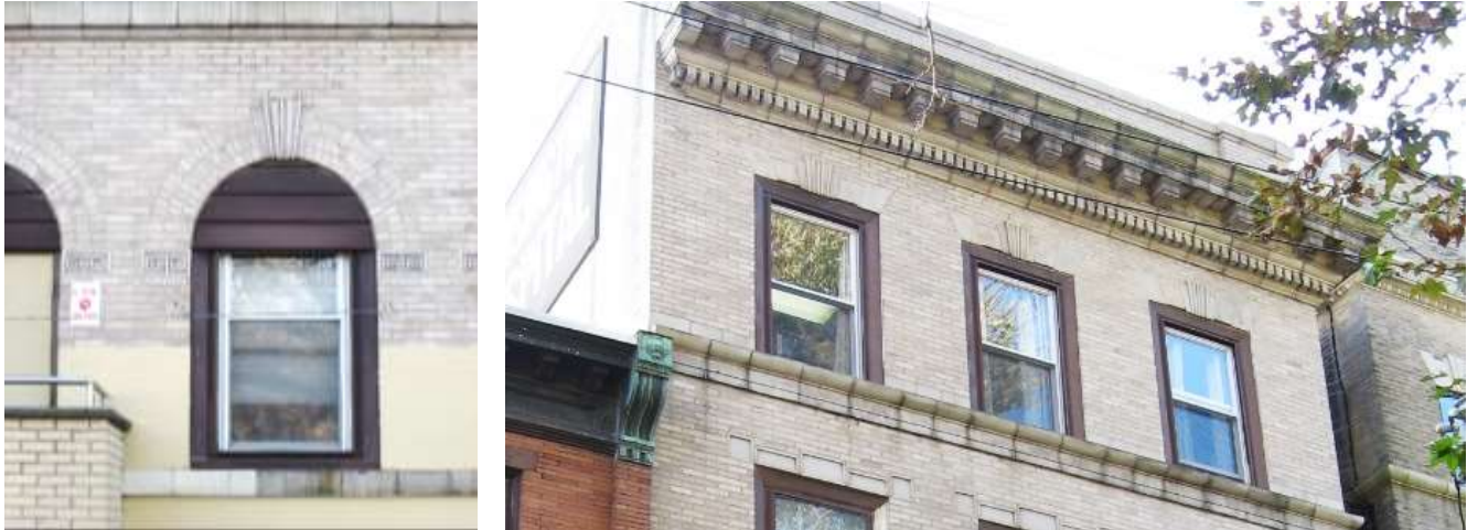
Figure 16: Left, first-floor window opening detail. Right, details of the cornice and parapet and ornament above 3 rd and 4 th -floor windows.
