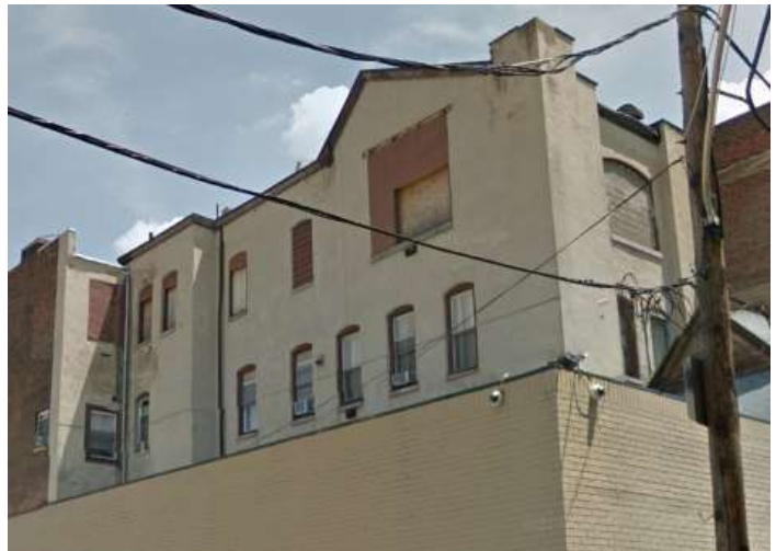
Figure 11: Left, the west elevation, and right, the west and south elevations, of the 1896 addition showing what had been large windows and the gabled upward extension of the roof for skylights, both for illumination of the operating room.
