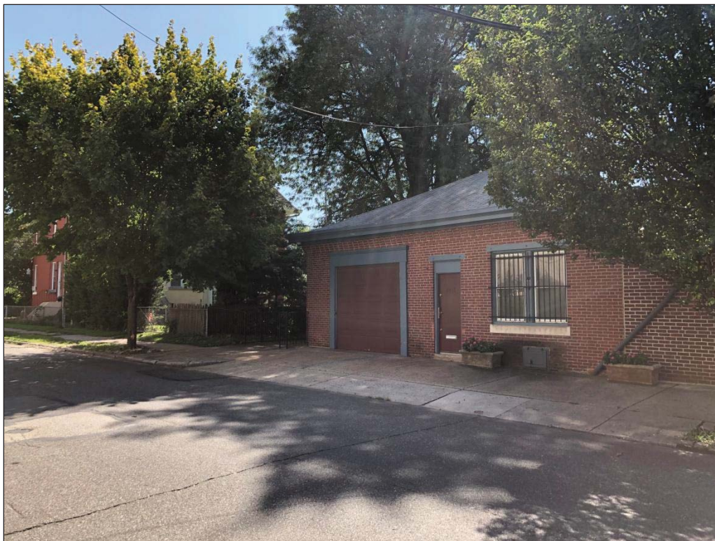
Figure 16: View of the north elevation of Laboratory building along Ditmas Street (2019). The Laboratory was constructed in close proximity to Frank Shuman's house. In this photograph, the house is visible on the left side of the image. The small addition is visible on the right side of the photograph. The division between the original building and the addition is visible by the difference in brick and mortar color.
