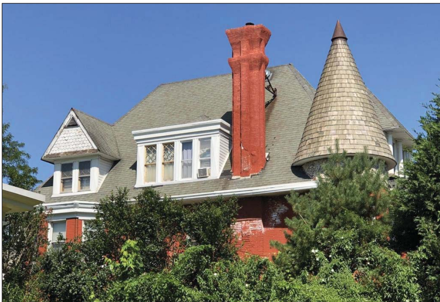
Figure 11: Roof above the south elevation (2019). Surviving details such as fish scale shingles, diagonal muntins, slate shingles, and a decorative frieze are visible on the south elevation.
