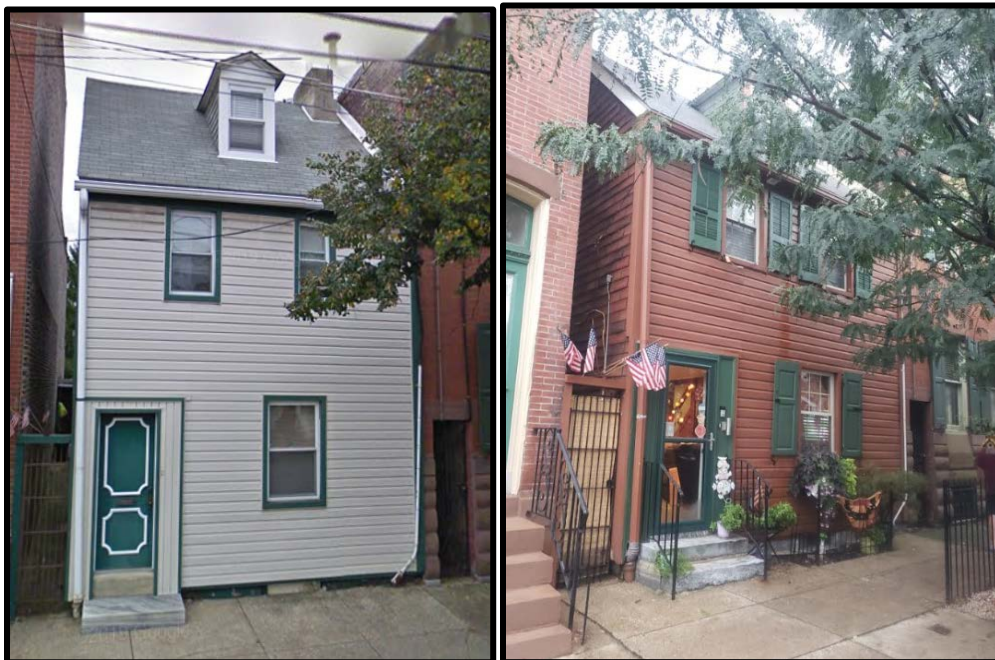
Figures 20 and 21. The above photographs show 1112 Marlborough Street before (left) and after restoration. The frame dwelling is a great example of what can be done to restore a period appearance to a wooden house with some relaxed standards. While the windows and siding appear to be of faux materials, the overall appearance of the house after renovation (right) has a historic quality. The 2009 Google Street View photograph (left) shows a much more mundane view of 1112 Marlborough Street. By 2013, Google Street View shows that house had been renovated to its present appearance (photograph on right taken in 2019). This building also appears to be of a similar wooden house form and scale as the subject property.
