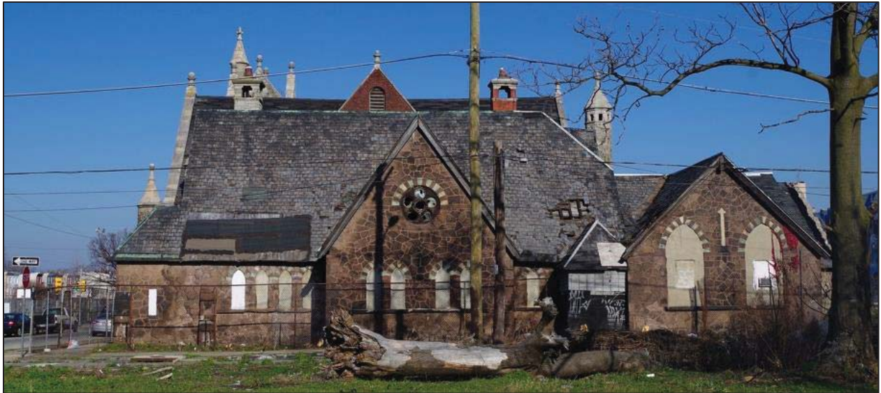
Figure 11: South elevation of the church complex showing the 1870 brownstone chapel and its 1876 addition to the east with pitched slate roof and the end gables of the narthex and transept. These portions of the property were used as a Sunday School, lecture room, and classrooms after the construction of the larger church in 1893 Photo by author.
