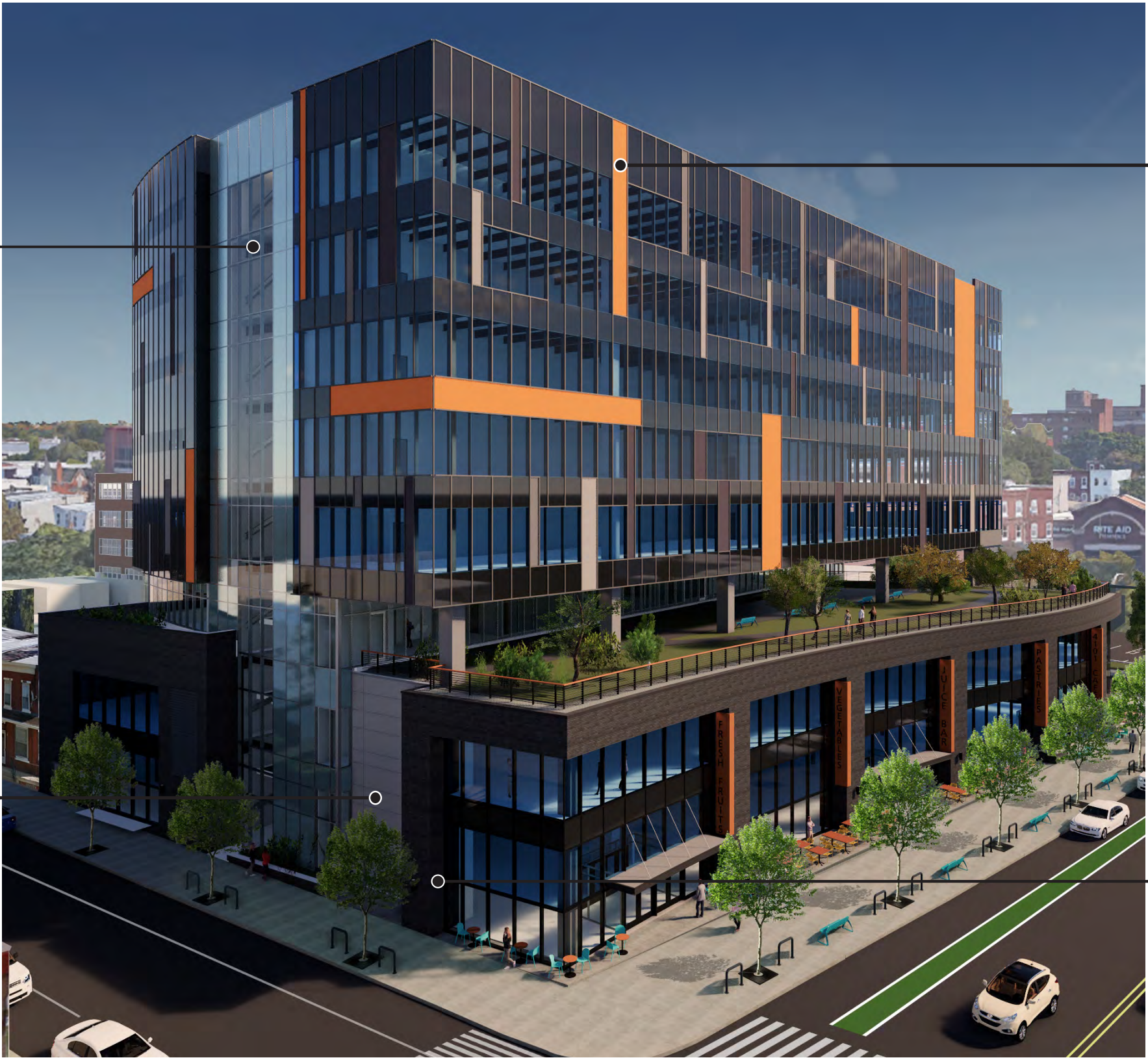
CURTAIN WALL ELECTROCHROMIC GLAZING & SPANDREL
