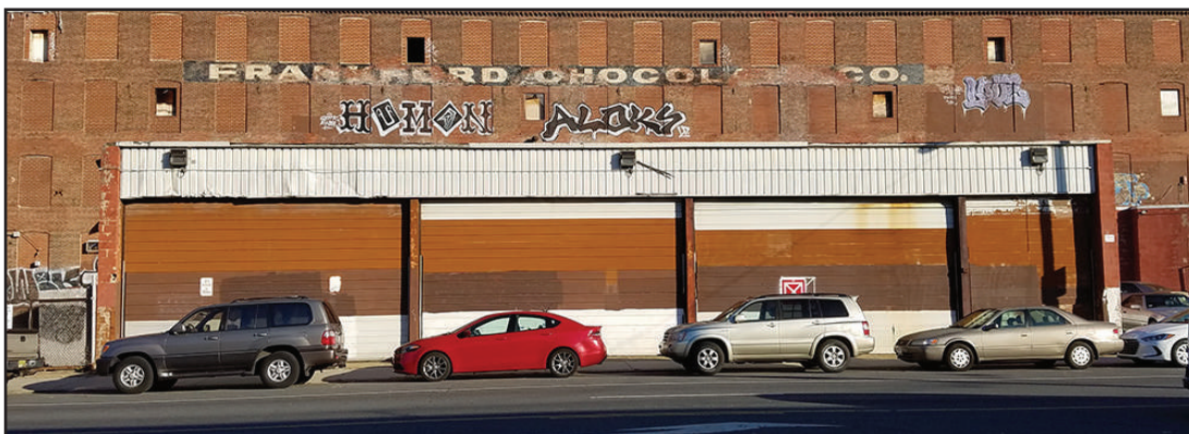
Figure 16: South elevation of 1967 Addition A. | Photo: Dennis Carlisle
