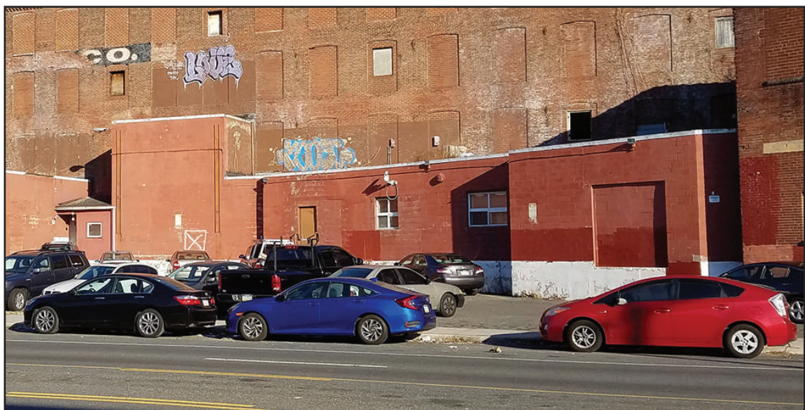
Figure 19: South elevation of 1967 Addition B. | Photo: Dennis Carlisle
