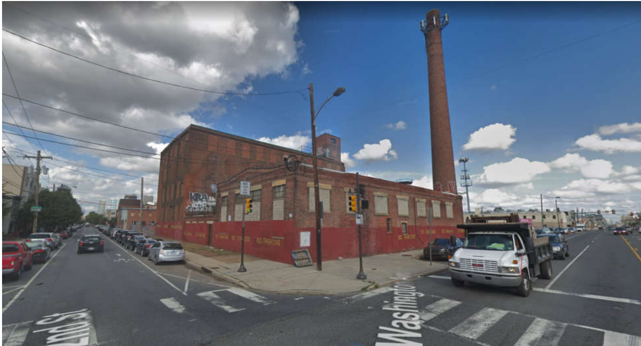
Figure 4. Looking to the northeast at the site from the corner of 22 nd Street and Washington Avenue, September 2018. Note that the smokestack was demolished after this photograph was taken.
