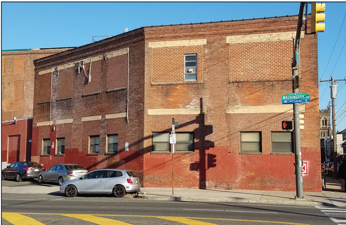
Figure 12: South elevation of 1912 Addition C | Photo: Dennis Carlisle
