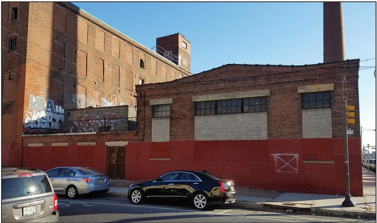
Figure 7: West elevation of the 1917 addition. | Photo: Dennis Carlisle
