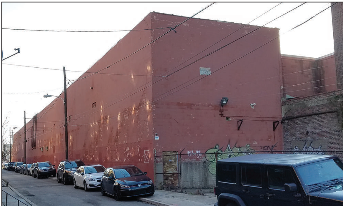
Figure 21: West and north elevations of the 1968 addition. | Photo: Dennis Carlisle
