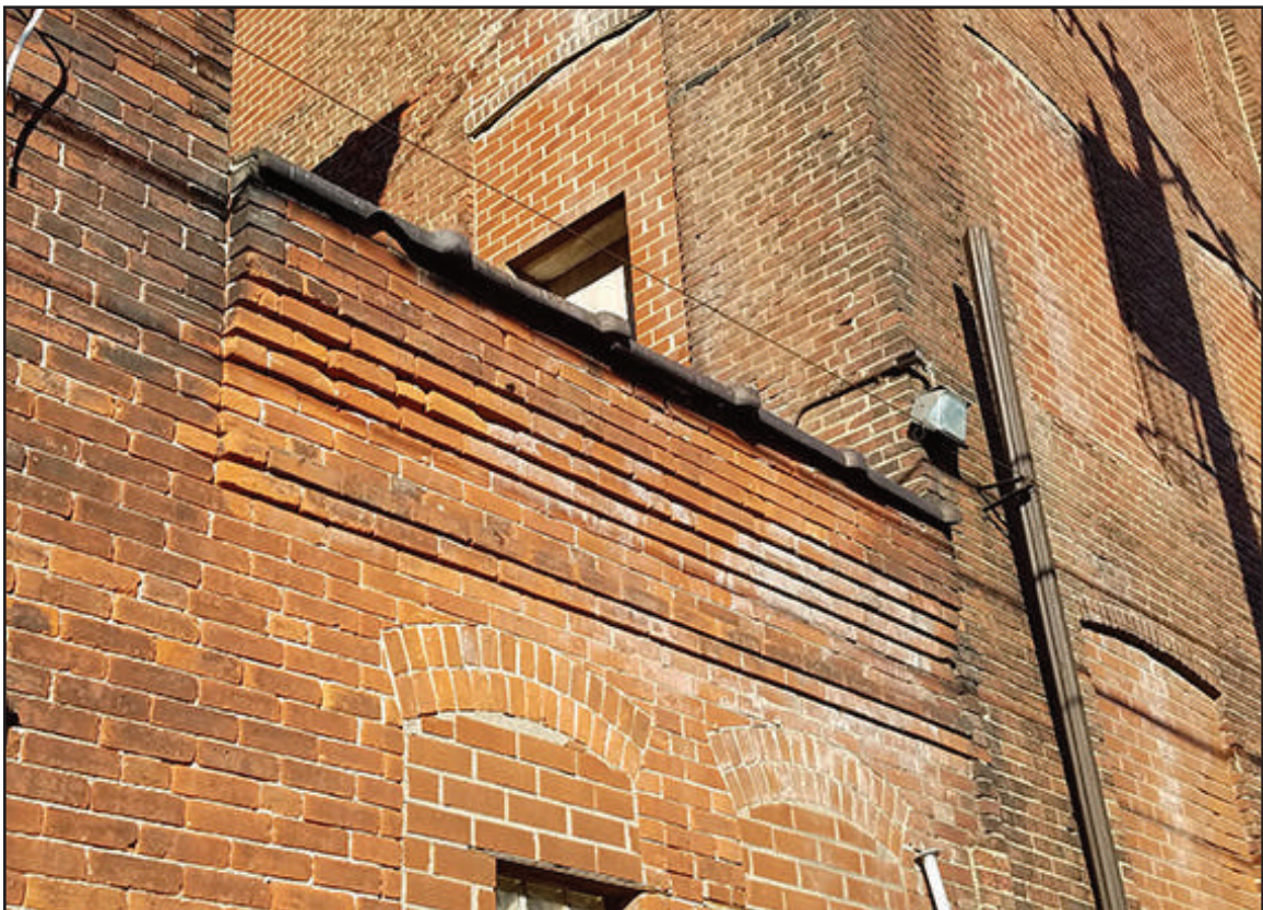
Figure 14: Detail of brick corbeling and terra cotta coping. | Photo: Dennis Carlisle
