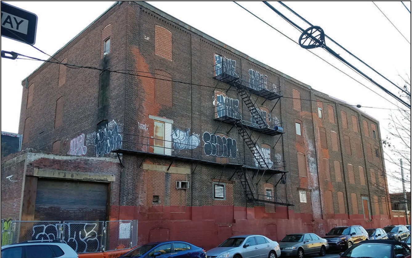
Figure 6: West and south elevations of the 1883 addition. | Photo: Dennis Carlisle
