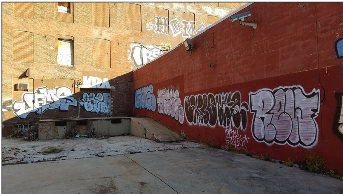
Figure 18: West elevation of 1967 Addition A. | Photo: Dennis Carlisle
