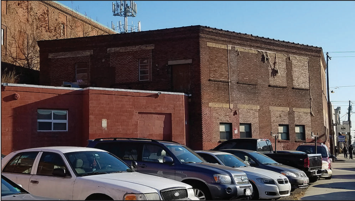
Figure 11: Southwest and west elevations of 1912 Addition C. | Photo: Dennis Carlisle
