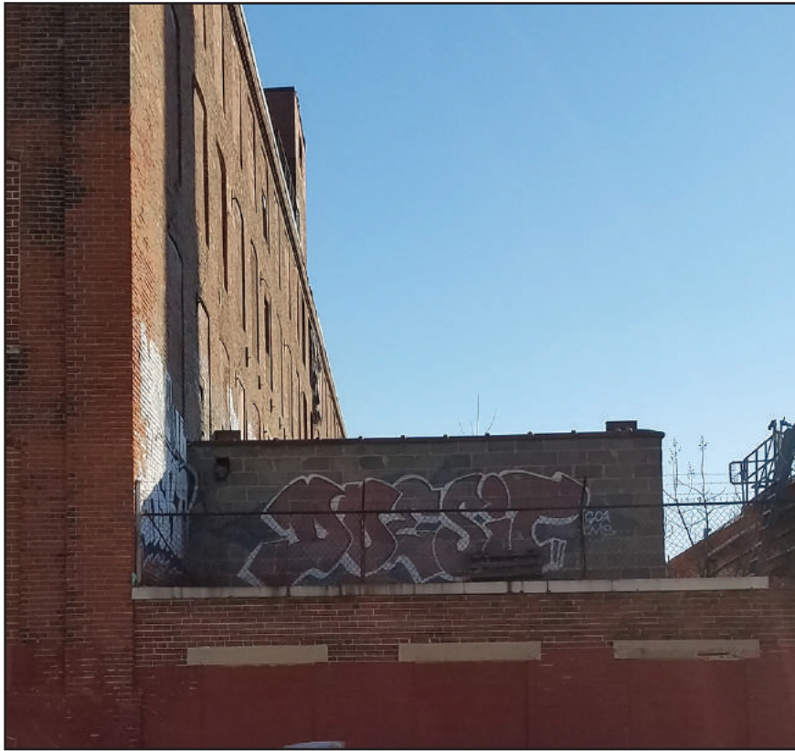
Figure 15: West elevation of the 1964 addition. | Photo: Dennis Carlisle
