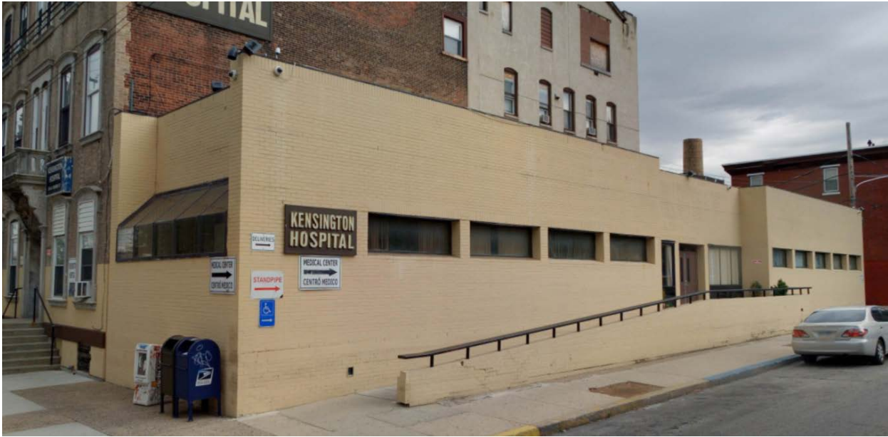
Figure 23: The 1978 outpatient clinic addition, viewed from the intersection of Diamond Street and N. Mascher Street. Source: Cyclomedia, 2018.
