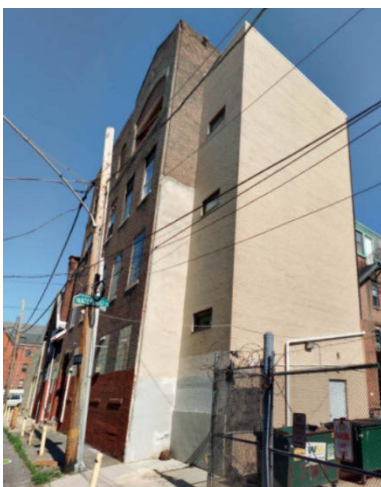
Figure 20: The east elevation of the Maternity Ward building features a non-historic stair tower .Source: Cyclomedia, 2018.
