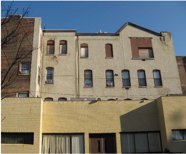
Figure 11: Left, the west elevation, and right, the west and south elevations, of the 1896 addition showing what had been large windows and the gabled upward extension of the roof for skylights, both for illumination of the operating room.
