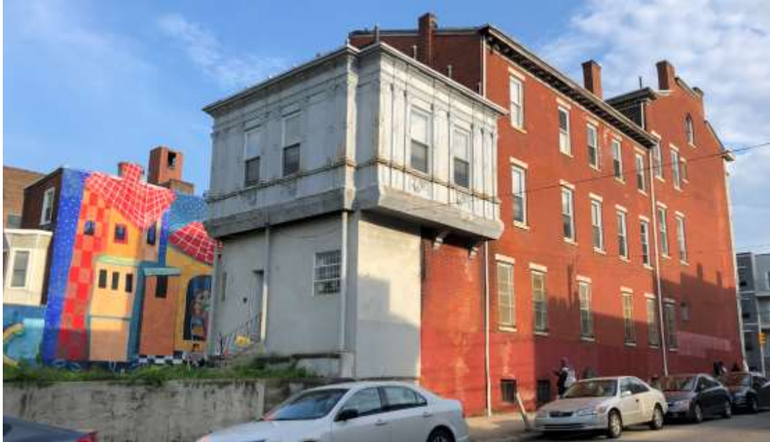
Figure 4: Looking southeast at the rear (north) and west side elevations, May 2019.
