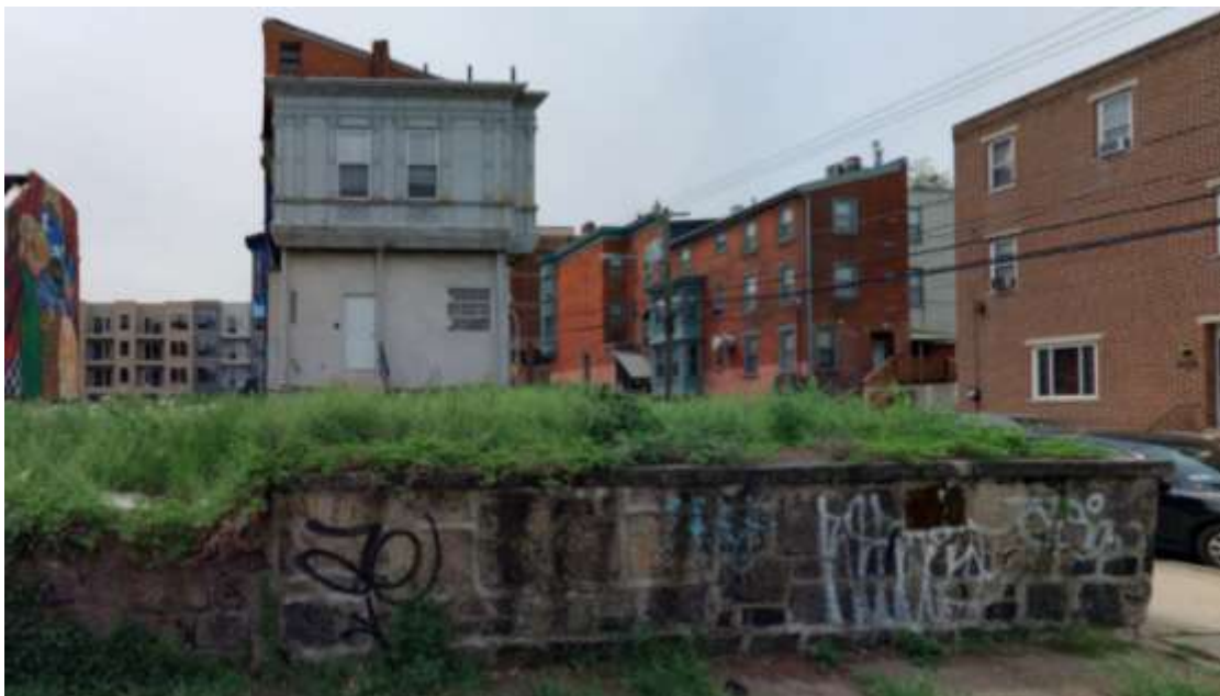
Figure 5: View south towards the rear, north elevation of the property from Flora Street, May 2019.
