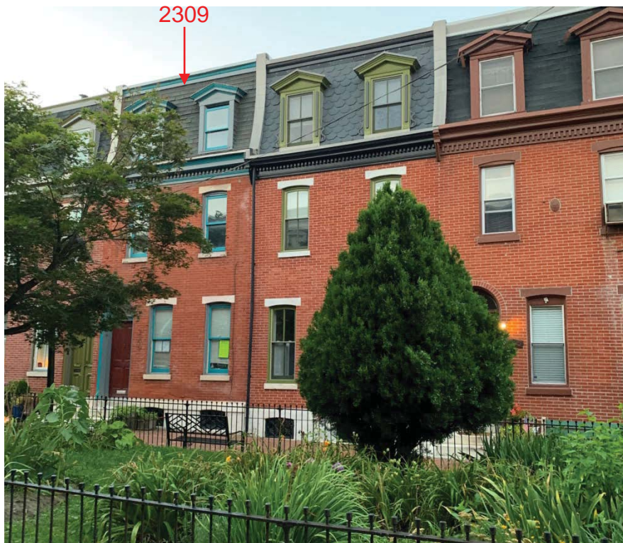
Figure 2: Front façade of 2309 St. Albans Street, 2019.
