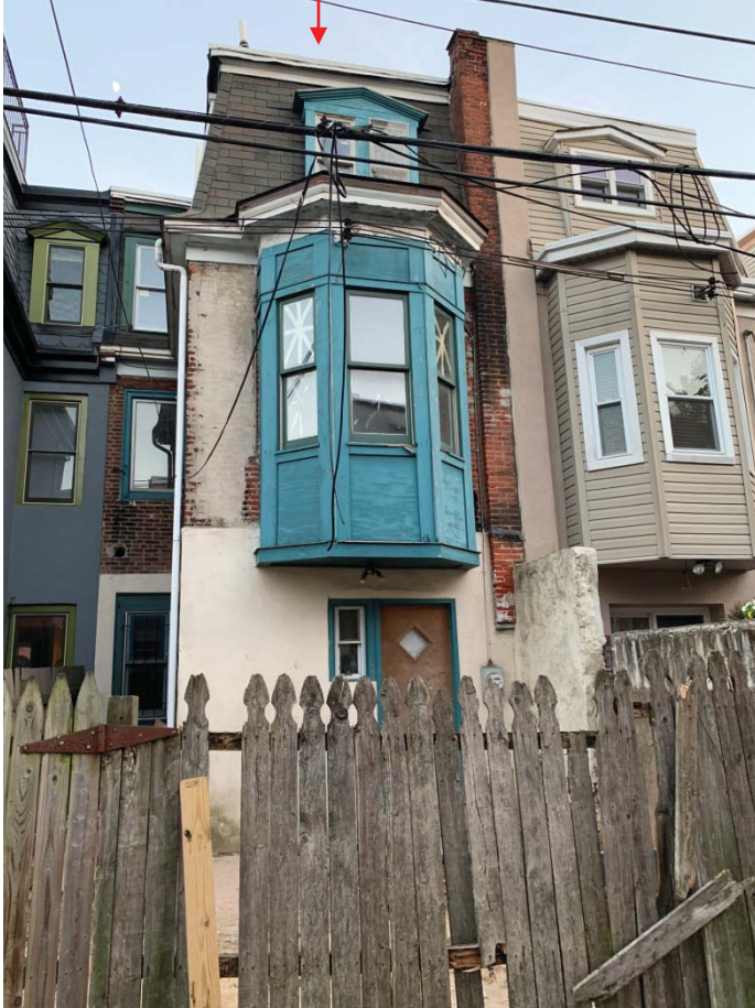
Figure 3: The rear of 2309 St. Albans Street, 2019.
