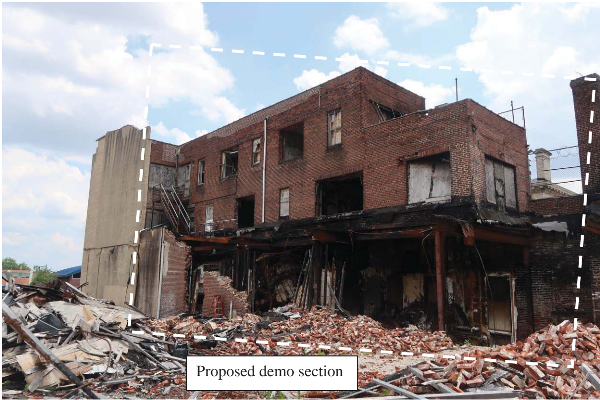
Photo No. 8. The front (east) section of 1512-16 N. Broad Street, Philadelphia
