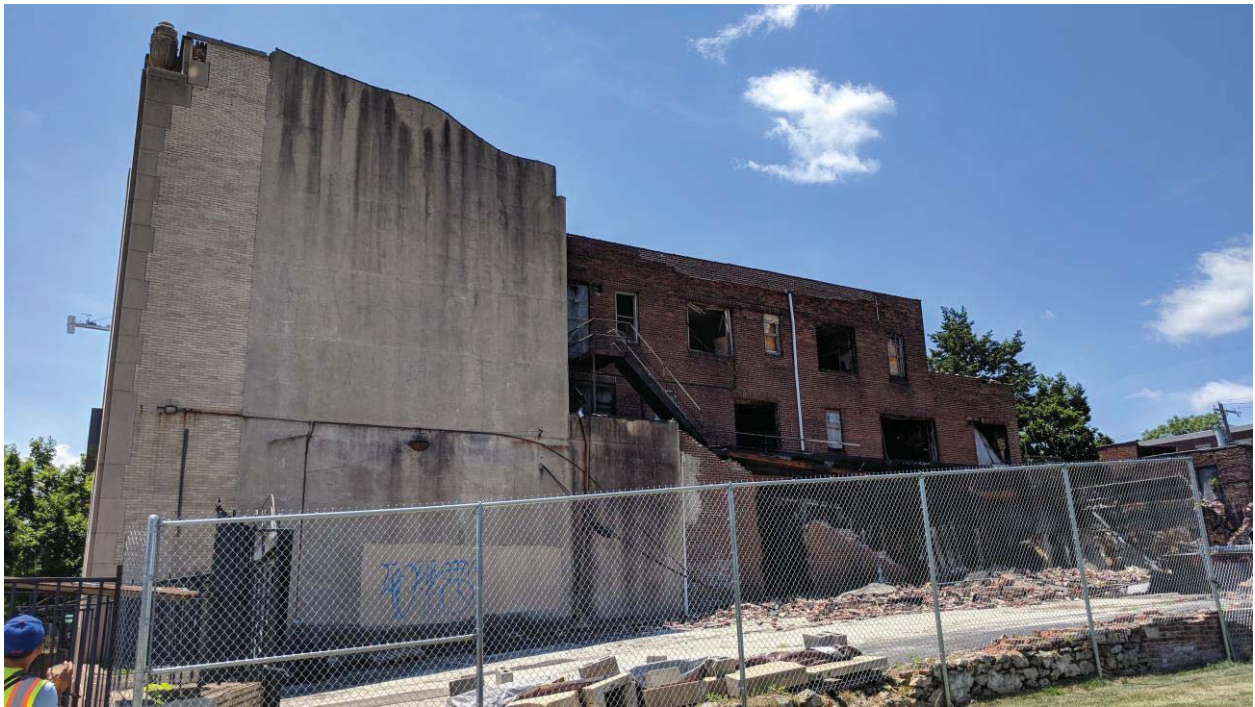
Photo No. 3. View of north facing side of building
