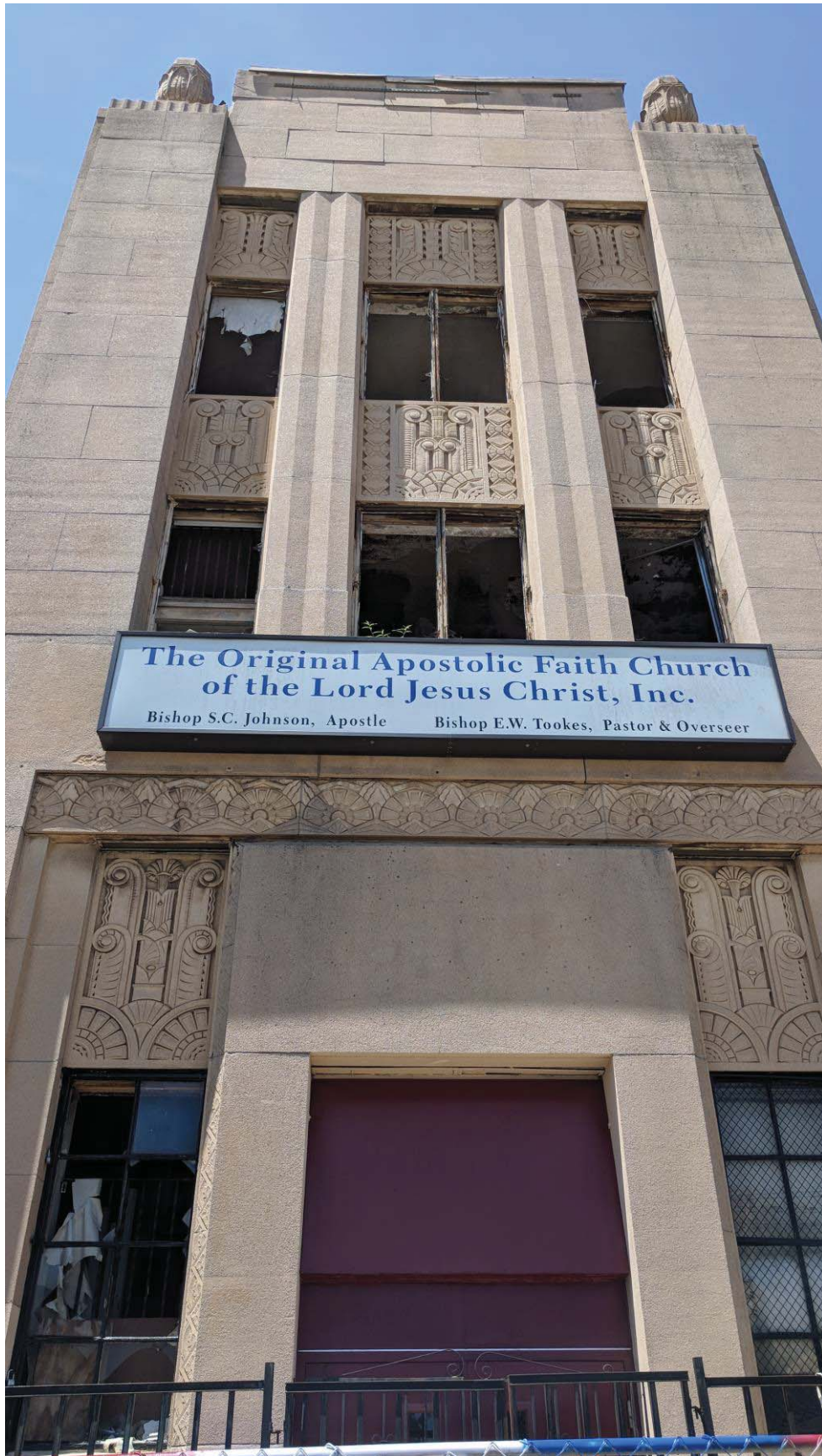
Photo No. 1. Front view of 1512 N Broad Street, Philadelphia, PA 19121
