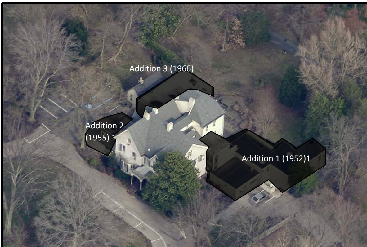
Figure 14. Looking northeast at the subject property, the non-contributing portion is highlighted in black—Additions 1, 2, and 3. Source: Atlas, City of Philadelphia, 2018.
