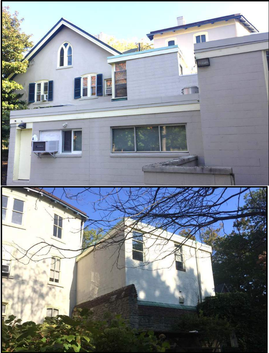
Figure 16. Top: The southwest elevation of the subject property with Addition 1 in the foreground. Bottom: The rear elevation of the subject property, Addition 3 is the two-story block building in the foreground at center and is considered non-contributing. The three-story building of left and the stone wall beneath the Addition 3 are both contributing. Source: Oscar Beisert, 2018.
