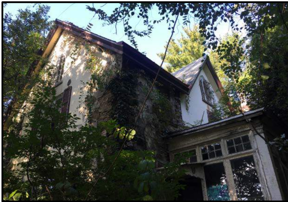
Figure 21. The southeast and rear (northeast) elevations of the cottage, stable, or residence and carriage house-stable building that was formerly associated with the subject property. Source: Oscar Beisert, 2018.
