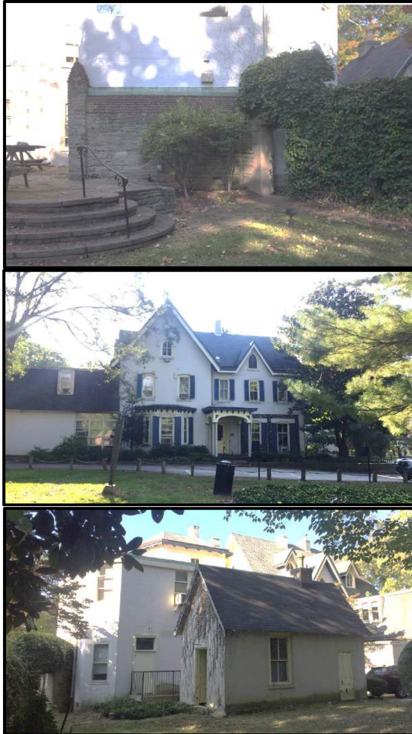
Figure 17. Top: Looking northwest at an old garden masonry wall, which is considered contributing, while Addition 3, the two-story block building above/behind it, is non-contributing. Center: Looking southeast, Addition 2 is considered non-contributing, located at the far left of this photograph. Bottom: Looking southwest, Addition 3, the two-story block building on left, is considered non-contributing, while the Shed in the foreground on right is considered contributing. Source: Oscar Beisert, 2018.
