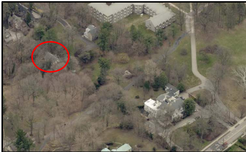
Figure 23. Looking southeast at the subject property. Source: Pictometry, City of Philadelphia, 2018.
