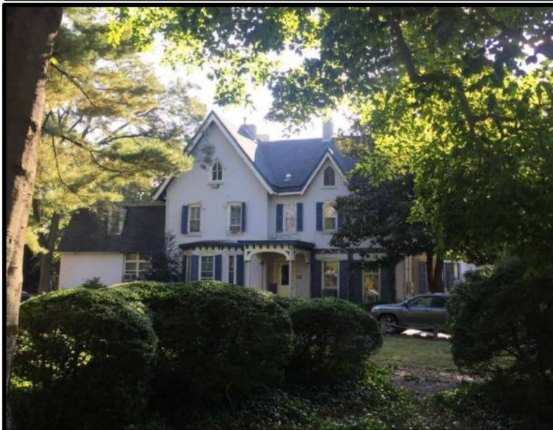
Figure 18. Top: “Design XX. Villa Farm House,” as illustrated in Andrew Jackson Downing’s The Architecture of Country Houses (1851). Bottom: The primary (northwest) elevation of the subject property. Source: Oscar Beisert, 2018.
