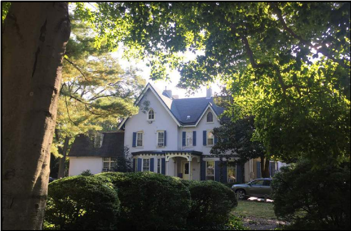
Figure 3. Top: The primary (northwest) elevation and yard of the subject property. Bottom: The primary (northwest) elevation of the subject property. Source: Oscar Beisert, 2018.
