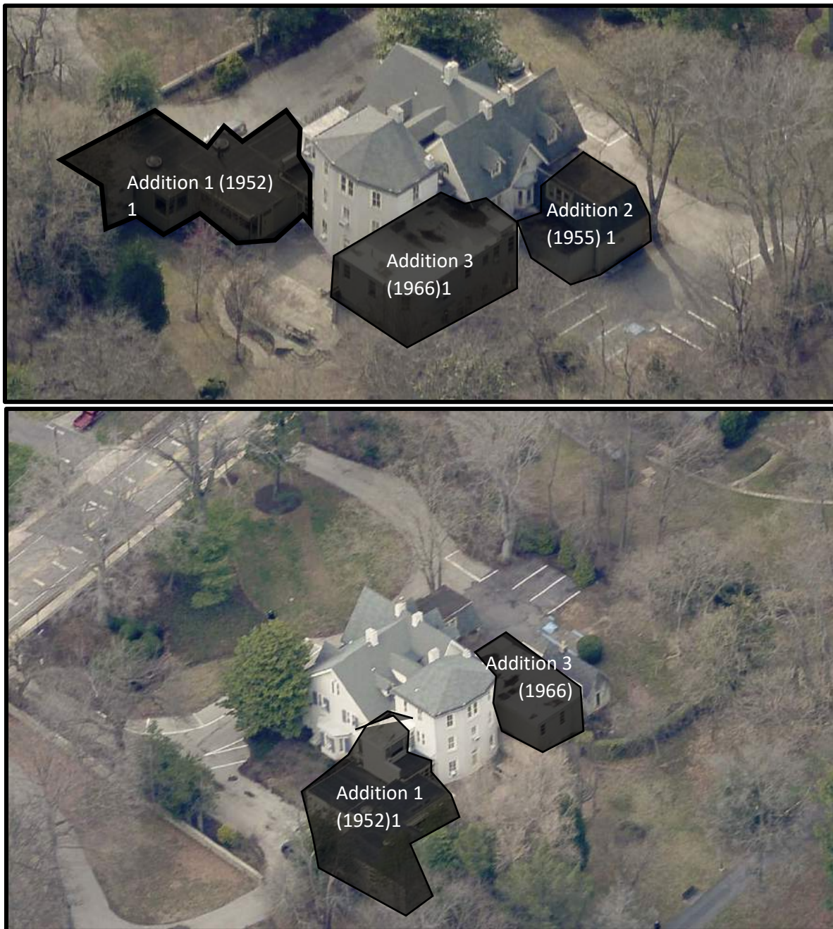
Figure 15. Top: Looking southwest at the rear of the subject property, the non-contributing portions are highlighted in black—Additions 1, 2 and 3. Bottom: Looking northwest at the rear elevation of the property, the non-contributing portions are highlighted in black—Additions 1 and 3. Source: Philadelphia Atlas.
