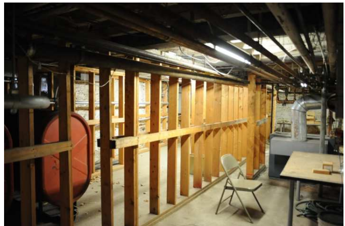
Smith house emergency shoring in basement under added partitions on first floor to reduce spans of termite damaged timbers
