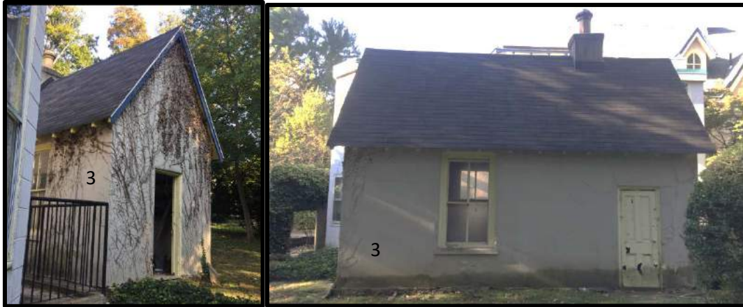
Figure 13. The numbers used in the photographs above correspond with the list of “Landscape Features” at the center of the previous page. Left: Looking northwest at the rear elevation of the shed building in the Gothic Revival style. Right: Looking south at the side (northeast) elevation of the shed building. Source: Oscar Beisert, 2018.
