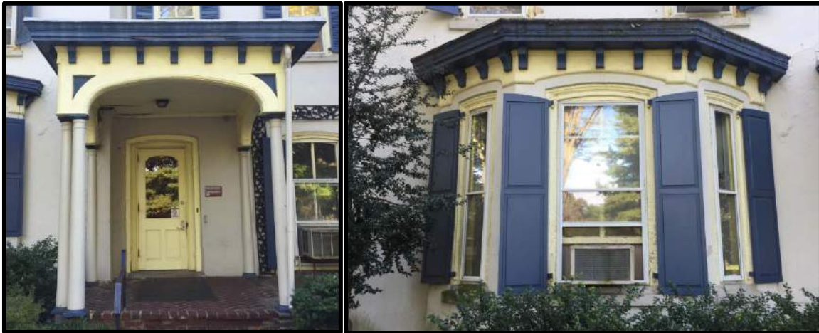
Figure 7. Left: The entrance porch and its bracketed treatment within the primary (northwest) elevation of the subject house. Right: The bay window and its bracketed treatment within the primary (northwest) elevation of the subject house. Source: Oscar Beisert, 2018.
