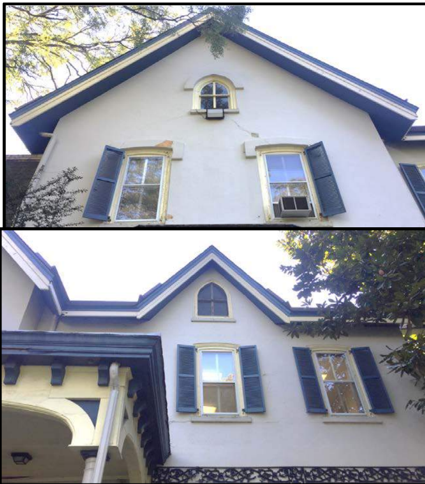
Figure 5. Top: The upper floors of the larger gable end within the primary (northwest) elevation of the subject property. Note, the window, defined by the pointed arch, as well as the window hoods on both floors. Bottom: The smaller gable within the primary (northwest) elevation. Source: Oscar Beisert, 2018.
