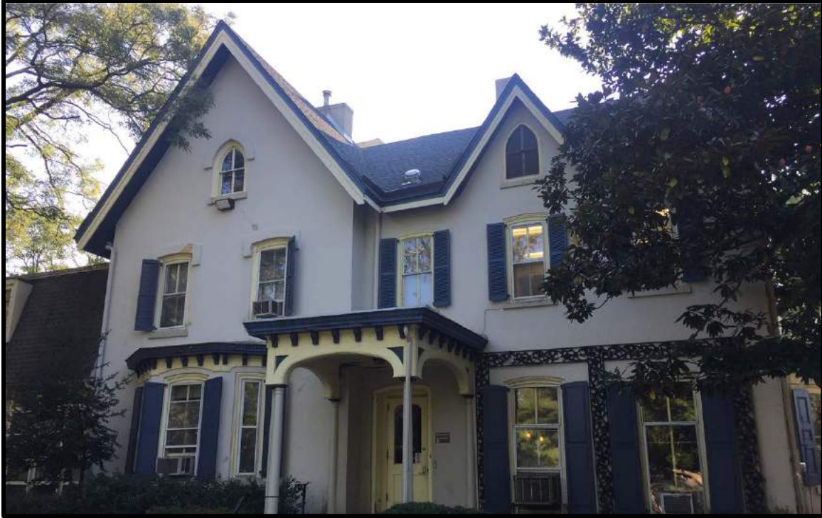
Figure 4. The primary (northwest) elevation. Source: Oscar Beisert, 2018.
