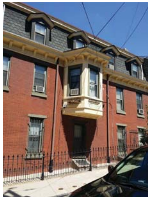
HP103.2 BAY WINDOW DETAIL. REMOVE ALL AL TRIM COVERM TYP SEE HP103.1
