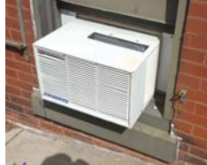
HP103.8 ONE OF MULTIPLE WINDOW A/C UNITS - REMOVE ALL EXISTING
