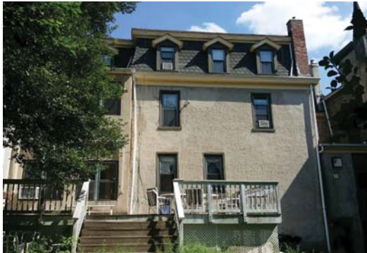
HP103.5 EXISTING REAR YARD ELEVATION- CLEAN & PATCH STUCCO TO REMAIN. NEW FIBERGLASS DOUBLE HUNG WINDOWS WITH EXG MTL TRIM
