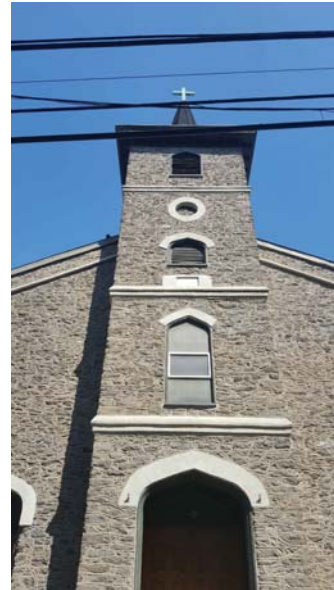
HP102.4 EXISTING CHURCH CONARROE ST ELEV. PAINT EXG WOOD TRIM. REMOVE EXG EXTERIOR PLEXIGLASS
