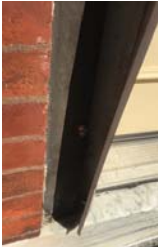
HP103.10 REMOVE METAL TRIM/ SILL/ HEAD AND REPLACEMENT WINDOWS ON CONARROE ST FACADE. REPLACE WITH ALUM CLAD WOOD WINDOWS AND BRICK MOULD TRIM. REPAIR AND PAINT EXG WOOD SILL AND LINTEL
