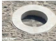
HP102.12/13 EXISTING ROUND CHURCH OPENING. REPLACE WITH NEW AL CLAD WINDOW WITH REPURPOSED STAINED GLASS. & AL CLAD TRIM. NEW ROUND WINDOWS SIMILAR.
