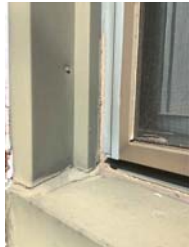
HP103.10 REMOVE METAL TRIM/ SILL/ HEAD AND REPLACEMENT WINDOWS ON CONARROE ST FACADE. REPLACE WITH ALUM CLAD WOOD WINDOWS AND BRICK MOULD TRIM. REPAIR AND PAINT EXG WOOD SILL AND LINTEL
