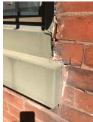
HP103.10 REMOVE METAL TRIM/ SILL/ HEAD AND REPLACEMENT WINDOWS ON CONARROE ST FACADE. REPLACE WITH ALUM CLAD WOOD WINDOWS AND BRICK MOULD TRIM. REPAIR AND PAINT EXG WOOD SILL AND LINTEL
