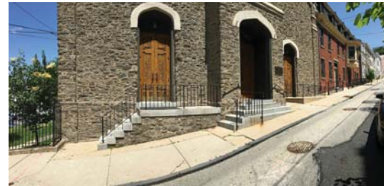
HP102.11 REPLACE (3) SETS OF EXISTING DOORS WITH paneled WOOD DOORS. PAINT EXG WD TRIM. SEE HP102.09 FOR TRANSOM INFO.
