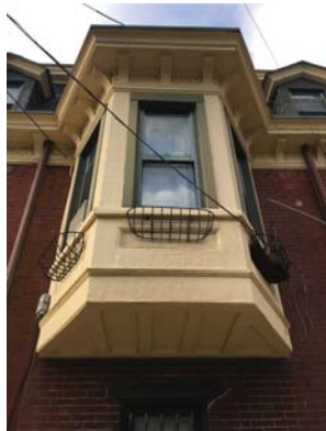
HP103.3 BAY WINDOW - REPLACE WINDOWS AND BRICK MOLD WITH ALUM CLAD. REMOVE METAL TRIM. RESTORE THE WOOD LINTEL AND SILLS & REPAIR.
