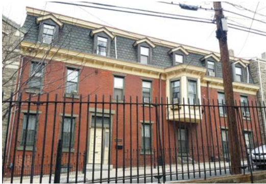
HP103.1 EXISTING CONARROE ST ELEV. REPOINT APPROX 30% TO MATCH EXG. REMOVE ALL METAL TRIM COVER. REPLACE ALL REPLACEMENT WINDOWS WITH DOUBLE HUNG DIVIDED ALUM CLAD WINDOWS & CLAD BRICK MOLD TRIM. EXG WD LINTEL AND SILLS TO BE REPAIRED & PAINTED.
