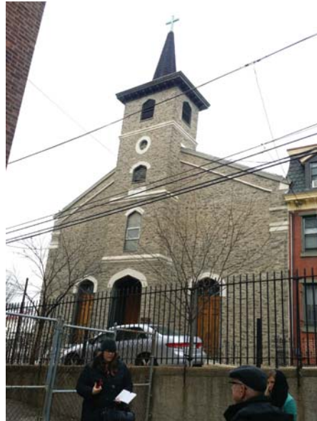
HP102.3 EXISTING CHURCH CONARROE STREET ELEV. REPLACE EXG WD VENTS WITH NEW CLAD VENTS. REPLACE ROUND WINDOW WITH CLAD, SEE SCHEDULE. REMAINDER OF WINDOWS, DOORS, TRANSOMS TO REMAIN. PAINT WOOD TRIM
