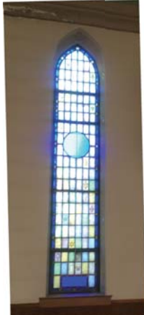
HP102.6/7 EXISTING CHURCH WINDOWS - REMOVE AND REPLACE WITH ALUM CLAD WOOD WINDOWS, ALUM CLAD BRICK MOLD. SEE ELEVATION. PORTIONS OF STAINED GLASS TO BE REUSED INSIDE PROJECT.
