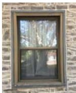
HP102.9 TYP EXISTING BASEMENT WINDOW - ALL BASEMENT WINDOWS TO BE REPLACED WITH ALUM CLAD AND CLAD BRICK MOLD
