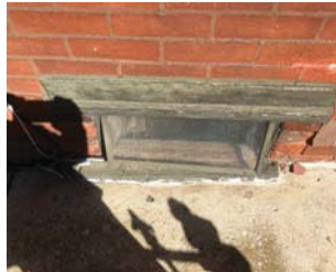
HP103.11 EXISTING REPLACEMENT WINDOW WITH EXPOSED WOOD LINTEL - THE ONLY OPG AT RECTORY WITHOUT METAL TRIM/COVER. REPAIR & PAINT.
