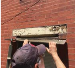
HP103.12 REMOVE ALL METAL TRIM COVERS - EXG WOOD TRIM BENEATH TO REMAIN. REPAIR, REPAINT, TYP
