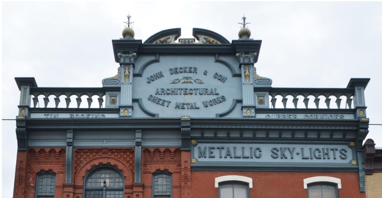
Figure 2: Cornice and parapet detail
