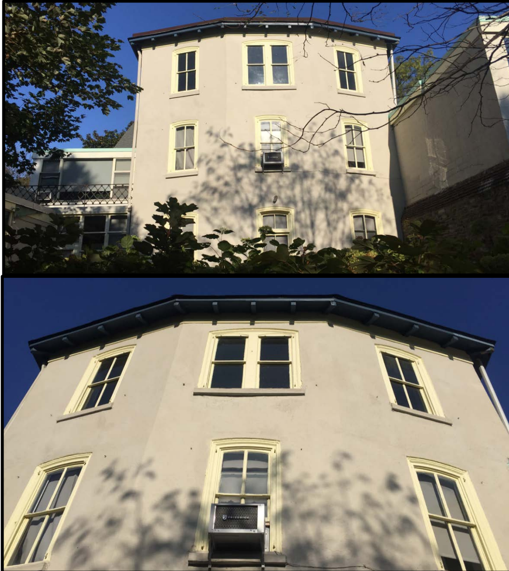
Figure 9. Top: The rear (southeast) elevation of the subject property. Note that the three-part façade features windows at each floor that are almost entirely original and/or early two-over-two wooden sash configuration. Bottom: The upper two floors of the rear (southeast) elevation. Source: Oscar Beisert, 2018.
