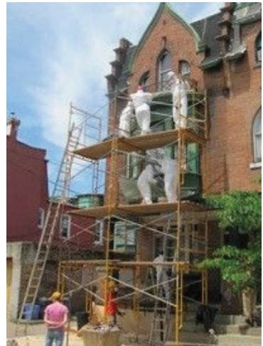
Habitat volunteers repair a facade.
