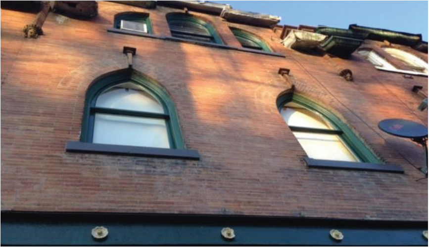
Facade restoration conformed to Historical Commission standards
