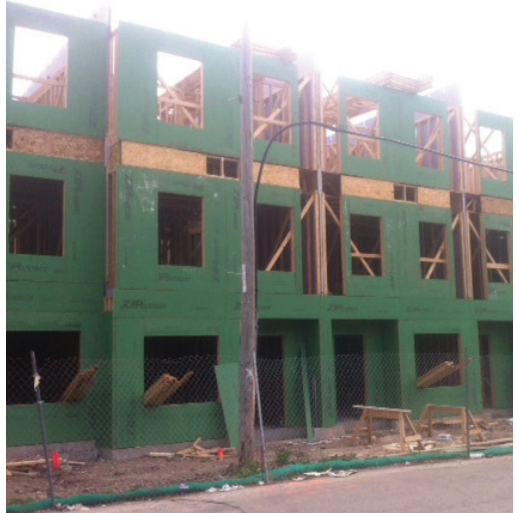
Grace Townhomes under construction.
