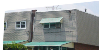
TYPICAL YORKTOWN MANSARD ASPHALT SHINGLE ROOF
