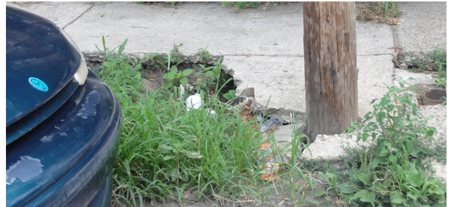
sidewalk cave-in likely caused by poor stormwater runoff issues
