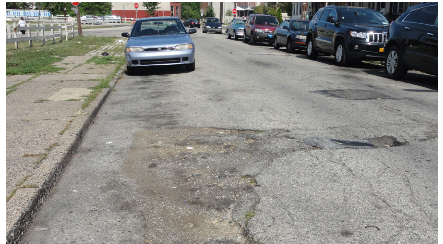
eroded street surface on wyalusing between 43rd and mantua
