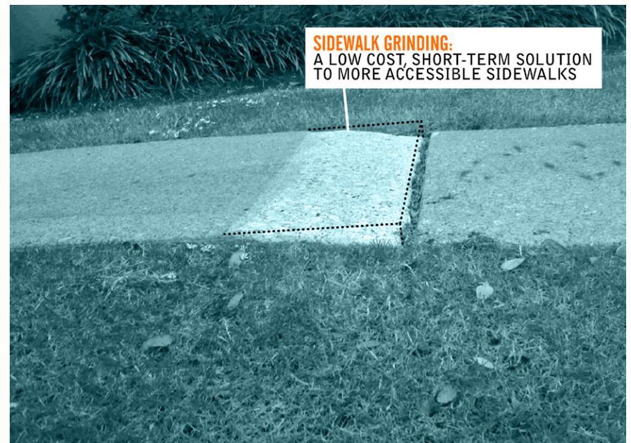
sidewalk griding can be a more cost effective way of fixing walkways
