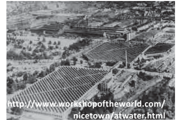
Aerial view of the Atwater Kent Radio Factory North and South Plant showing the “Super-Span Saw Tooth” roof trusses designed to incorporate natural light by Ballinger Architects and Engineers of Philadelphia in 1923.
