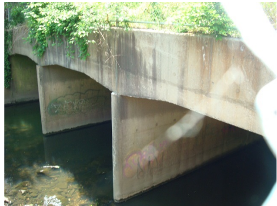
Figure 10: Existing 3 cell box culvert carrying Frankford Creek near Leiper Street
