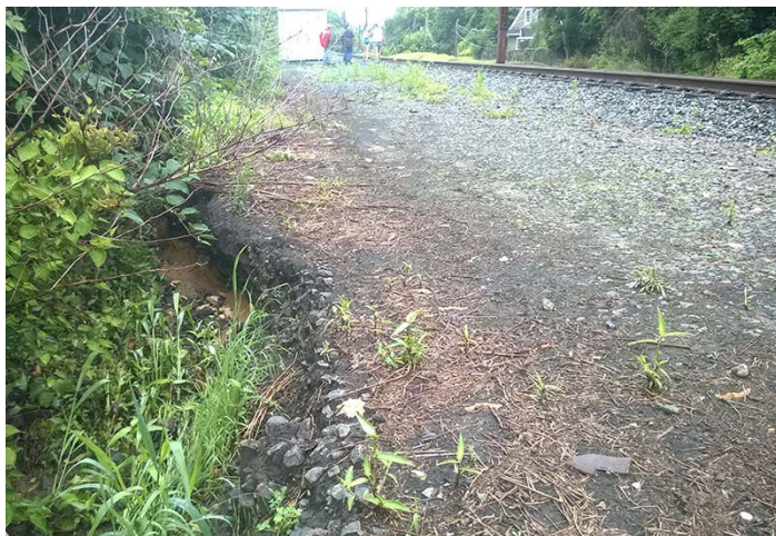
Erosion of railroad ballast caused by storm-water runoff
