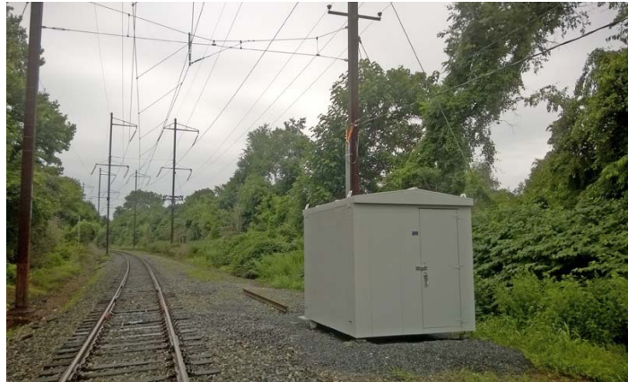
Signal building erected on vacant outbound track-bay, and catenary supports with guy wires, north of Woodbine Avenue
