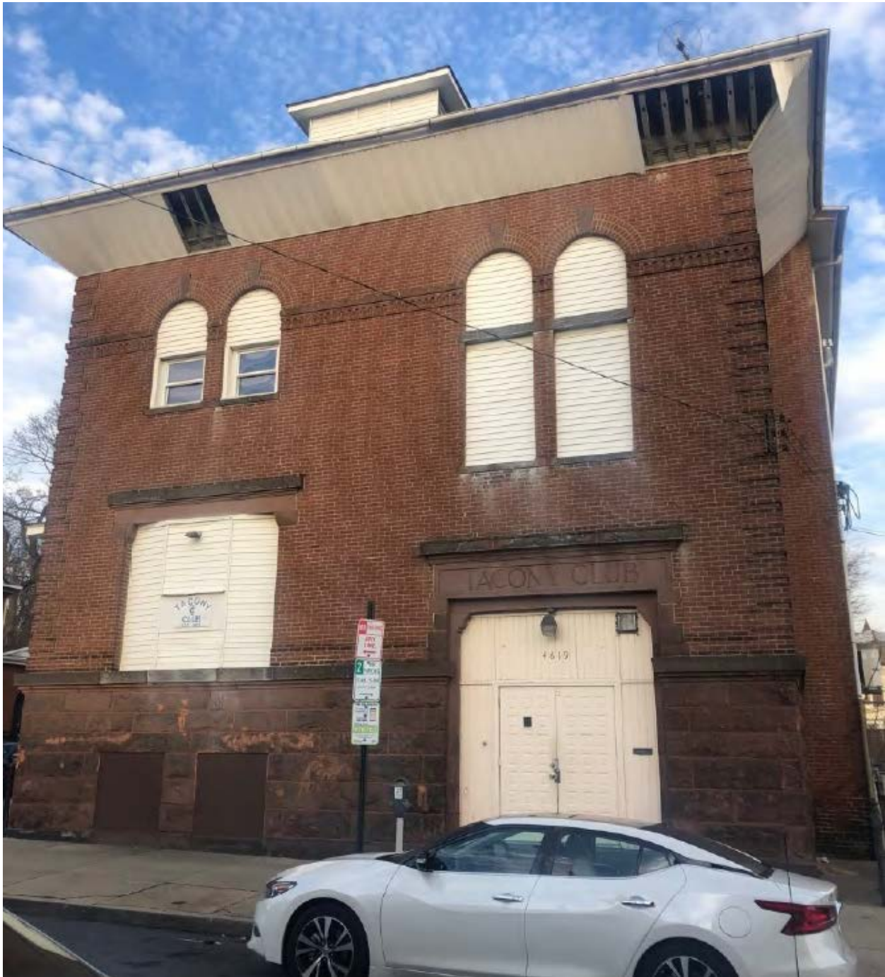
Figure 1. South façade along Longshore Avenue. Photograph by Alex Balloon, 2018.
