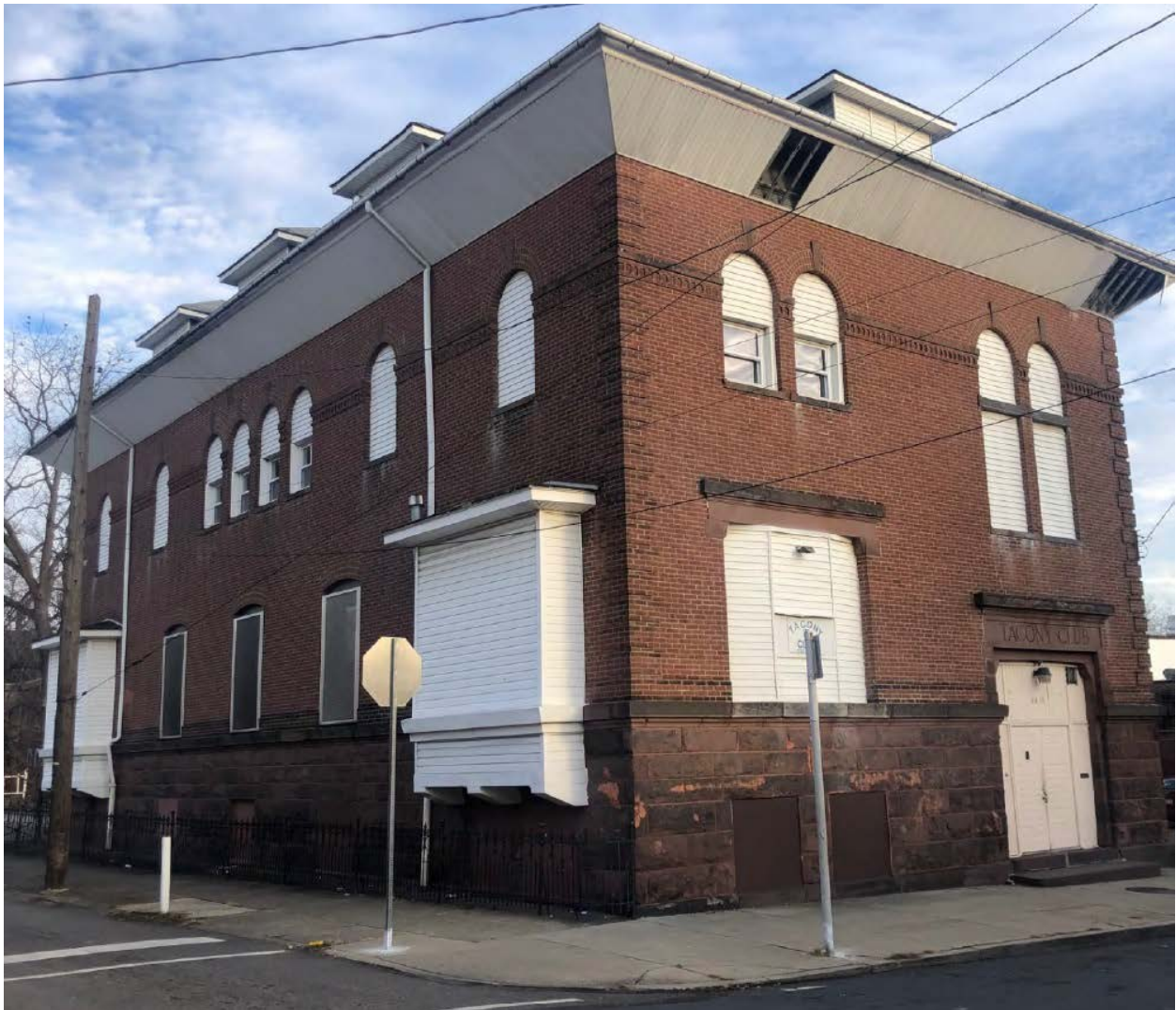
Figure 2. Southwest corner showing west façade facing Marsden Street and south façade facing Longshore Avenue. Photograph by Alex Balloon, 2018.
