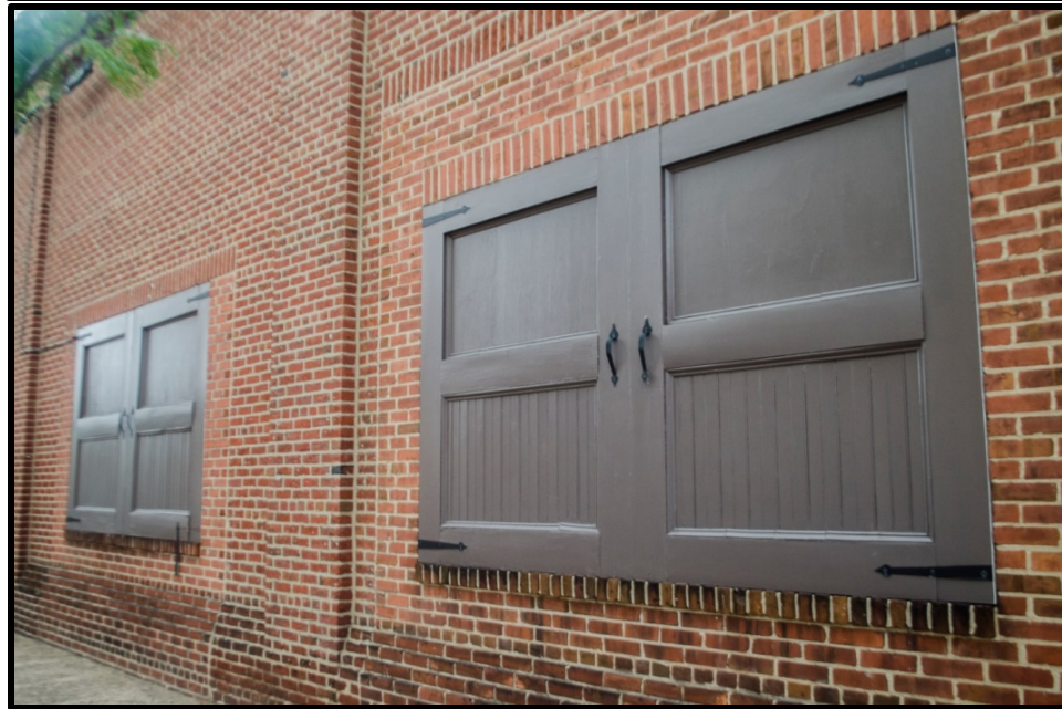
Top: looking north, the 41st Street Elevation of Buildings Nos. 2 and 3. Bottom: Looking southwest at the 41st Street Elevation of Building No. 3. Source: Annie Albert, 2017.
