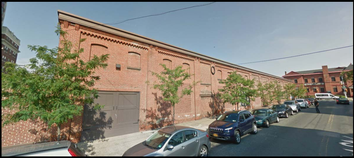
Top: Looking west at the 41st Street Elevation of Building 2. Source: Google Earth. Bottom: Looking northwest at the 41st Street Elevation of Building No. 2. Source: Google Earth.
