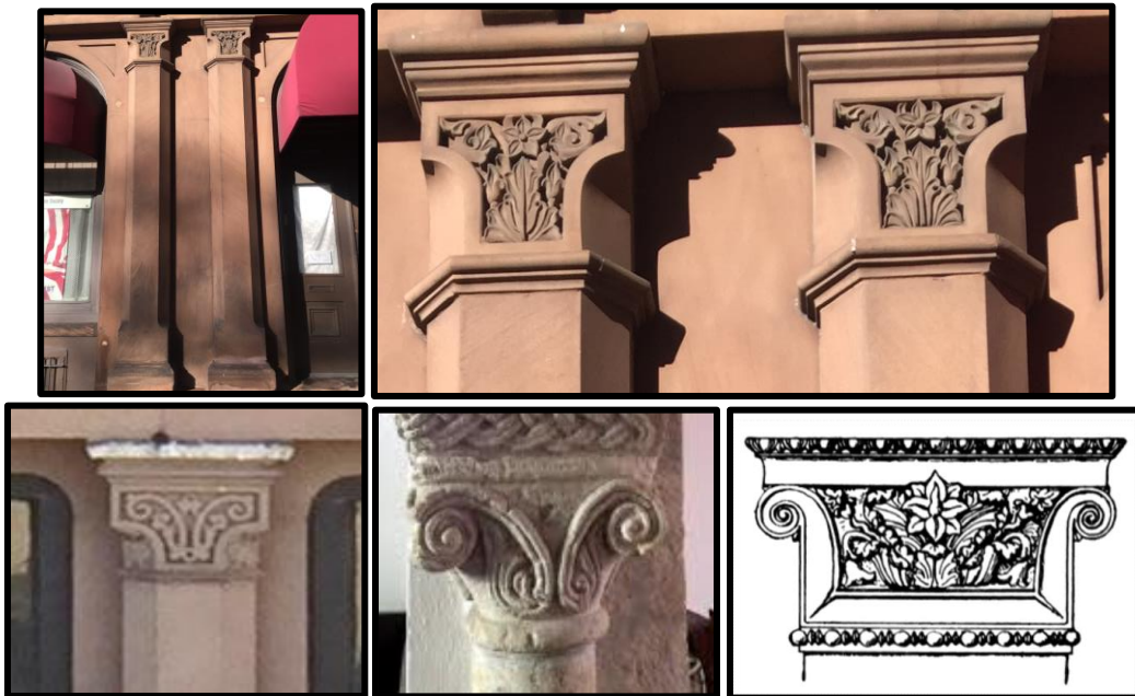
Figure 19: Top Left: Octagonal pilasters of the first floor, side (east) elevation of The Bible House at the northwest corner of Seventh and Chestnut Streets. Source: Oscar Beisert, 2018. Top right: Capitals, similar in form, but more elaborate in detail, of The Bible House. Bottom left: the capitals of the octagonal pilasters on the second floor of the subject property. Bottom center: a Norman period capital in Sussex. Source: http://sussexchurchez.blogspot.com/2011/02/st-james-selham.html . Bottom right: Capital with impost block, s. vitale. Source: Google.
