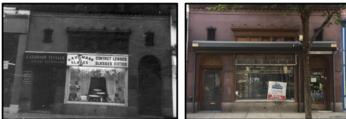
Figure 26: Left: The storefront of the primary (north) elevation, c. 1960-70. Source: Philadelphia Historical Commission. Right: the same view in 2018. Source: Oscar Beisert.
