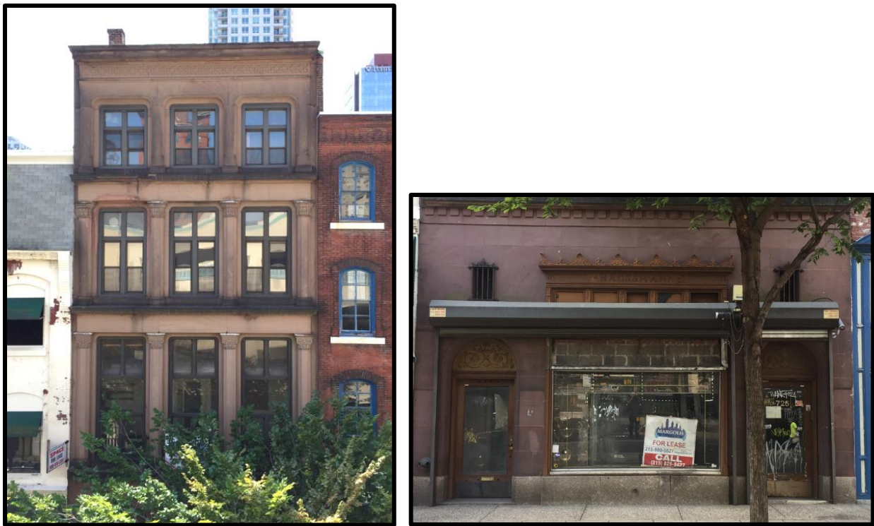
Figure 4: Left, the upper floors of the north elevation. Right, the storefront of the north elevation. Source: Oscar Beisert, 2018.
