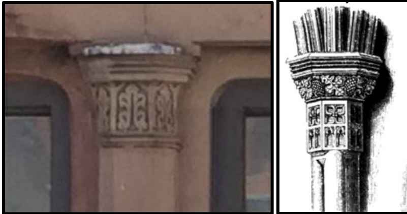
Figure 20: Left: the capital type, emulating the Perpendicular style, on the third floor of the primary (north) elevation of the subject property. A period Perpendicular style capital. Source: http://www.medart.pitt.edu/image/england/winchester/cathedral/text-willis/winc-willis-chapter3.html
