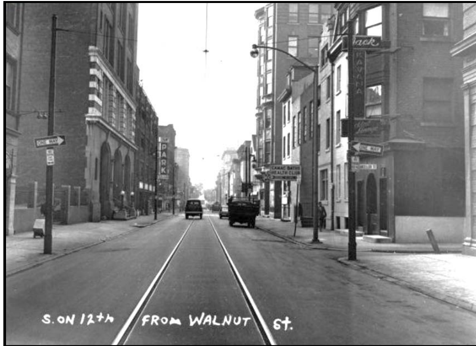
Looking south at the 200 block of South Twelfth Street below Walnut. The subject building at 200 South Twelfth Street is on the right. This photograph was taken in 1959. Source: DOR Archives.
