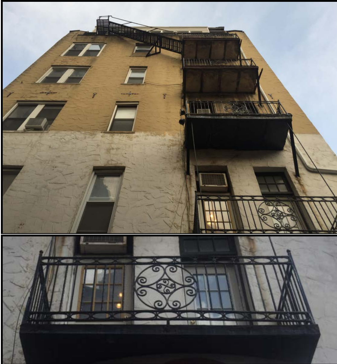
Top: Looking east at the upper floors of the S. Camac Street elevation, featuring wrought iron, Mission or Spanish-inspired balconies, and other discreet tile details. Bottom: A wrought iron balcony on the S. Camac Street elevation of the Camac Baths. Source: Oscar Beisert, 2018.
