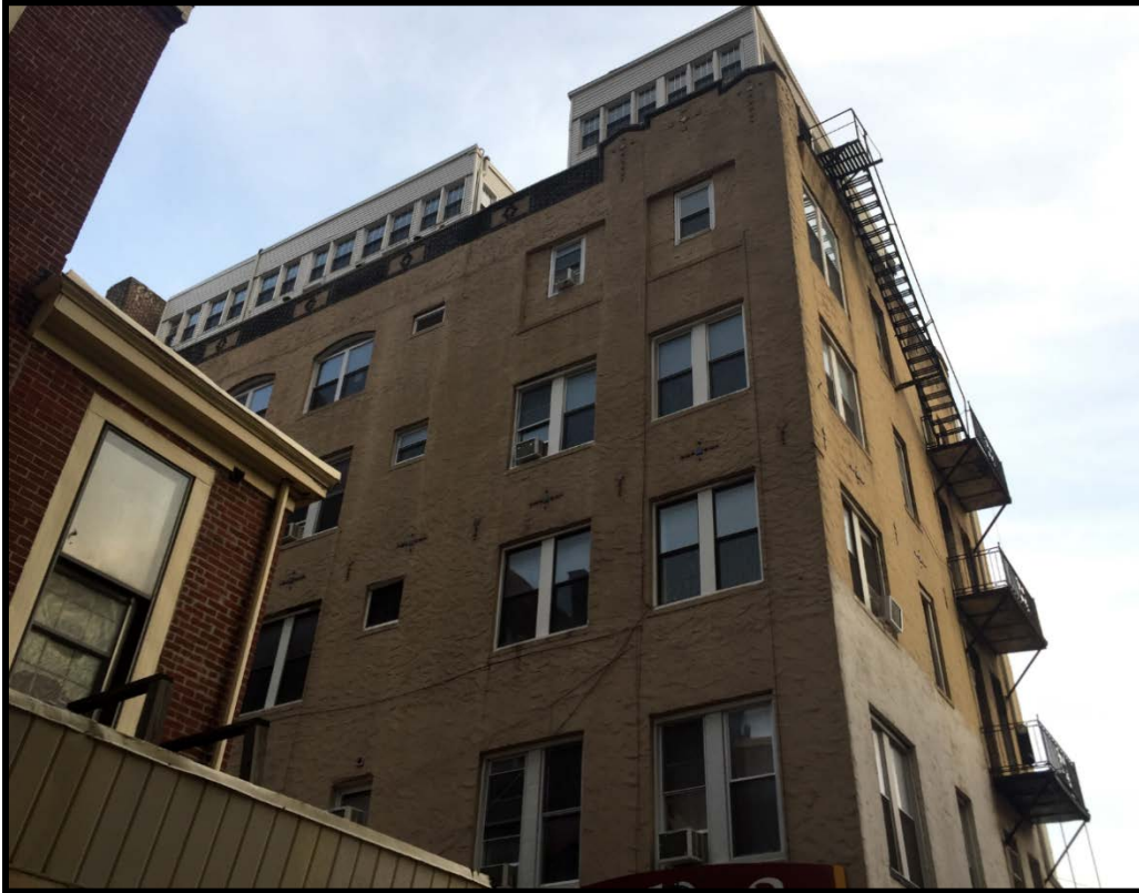
Looking southeast at the upper stories of the Camac Baths. Source: Oscar Beisert, 2018.
