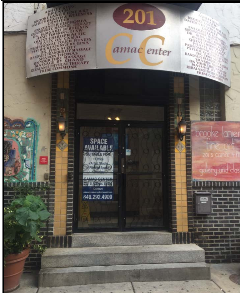
Top: The upper portion of the brick and tile surround at the primary, S. Camac Street entrance to the Camac Baths. Bottom: the lower portion of the brick and tile surround at the primary, S. Camac Street entrance to the Camac Bath. Note the original granite steps from 1907. Source: Oscar Beisert, 2018.
