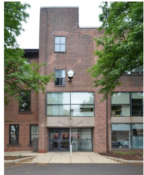
Figure 8: Contemporary entrance at west elevation.
