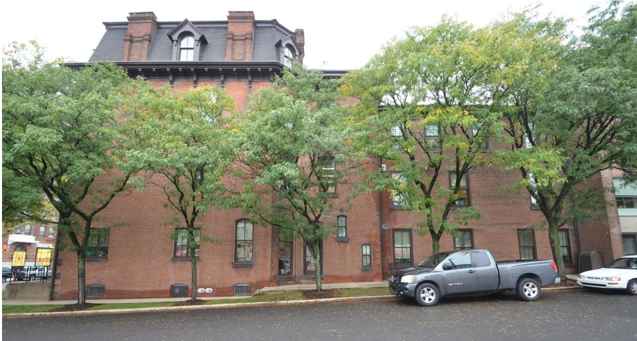
Figure 6: East elevation of 3825-27 Chestnut Street
