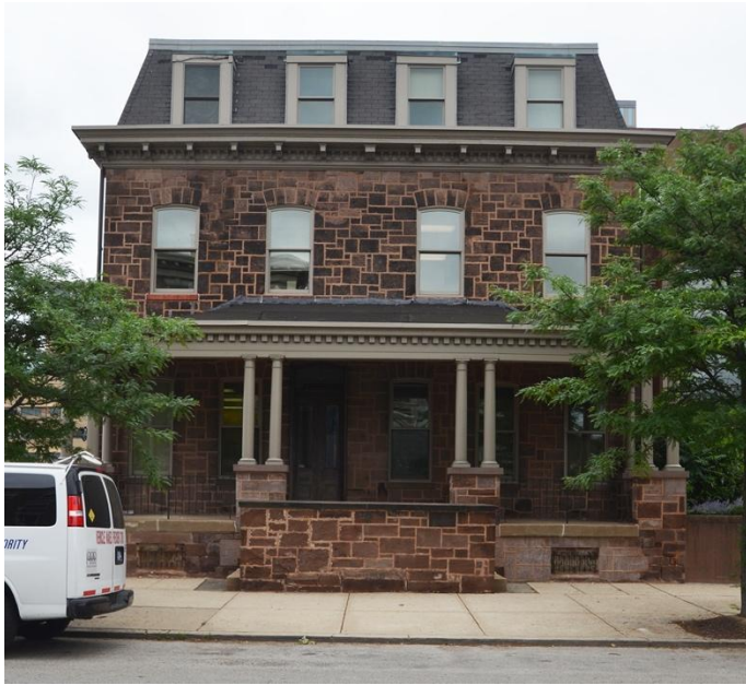
Figure 9: West (39 th Street) elevation of 19-21 S. 39 th Street
