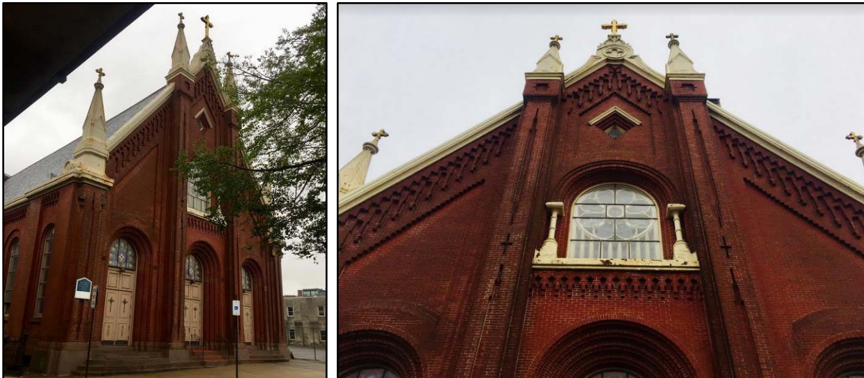
Figure 4: The primary (north) elevation of the Church of the Immaculate Conception along Allen Street. Source: Oscar Beisert, 2018.
