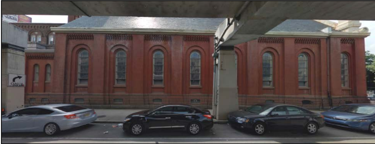
Figure 9: East elevation of the church along N Front Street. Source: Cyclomedia, 2018.
