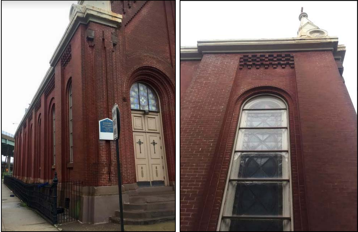
Figure 8: Details of the northeast corner of the church. Source: Oscar Beisert, 2018.
