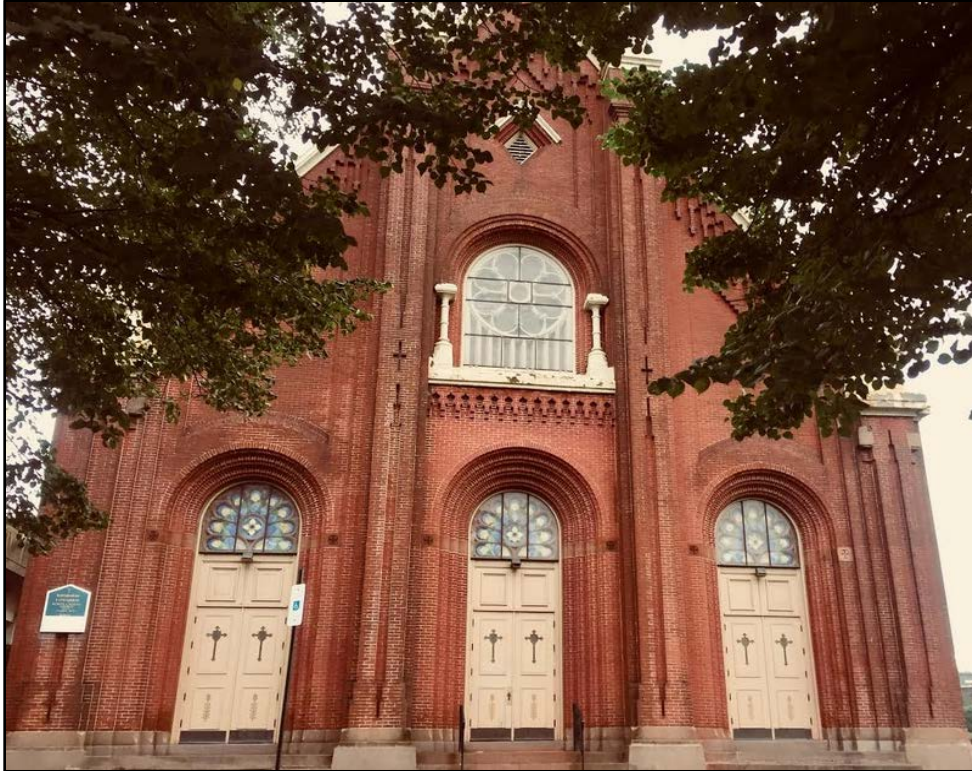
Figure 5: The primary, Allen Street elevation of the Church of the Immaculate Conception. Source: Oscar Beisert, 2018
