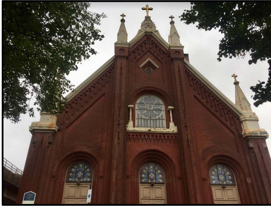
Looking south at the primary elevation of the Church of the Immaculate Conception. Source: Oscar Beisert, 2018.
