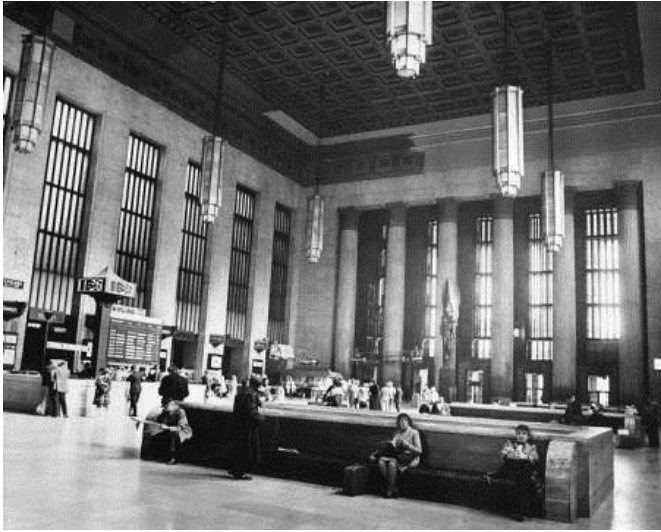
Figure 67: Main concourse in 1974. Philadelphia Evening Bulletin Collection, Temple University Libraries, Special Collections Resource Center
