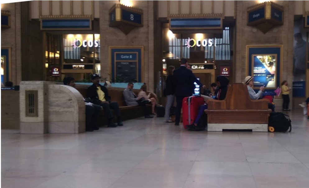
Figure 18 (top): Built-in oak benches with rounded stone end rests (left), oak waiting room benches on stone bases (right).
