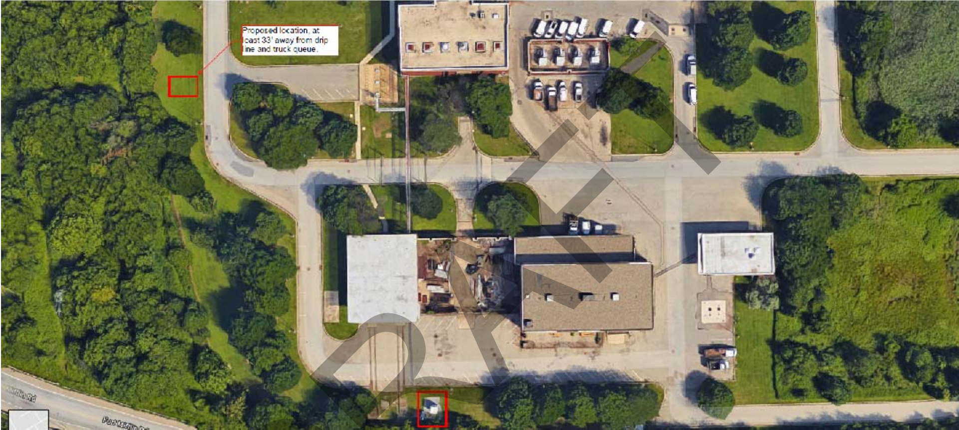
Figure 15 – SWA North Aerial View
