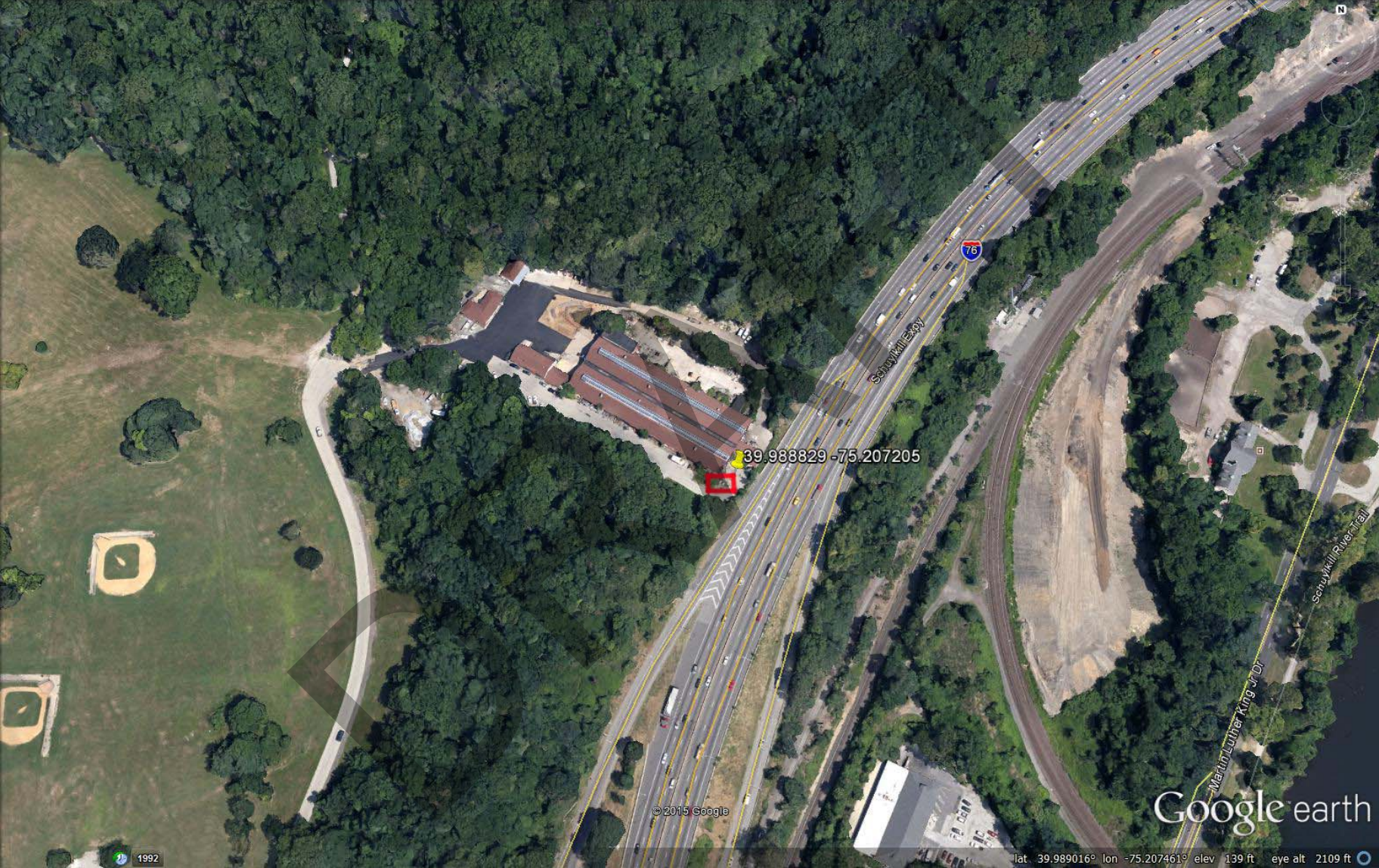
Figure 19 – MON North Aerial View
