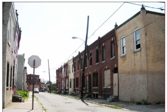
This stretch of almost exclusively vacant buildings is located on 45 th Street between Merion and Lancaster Avenues. The plywood doors and windows make accessing the properties easy. This is a public safety concern. This is also an example of street which is not wide enough to meet the Philadelphia Code
