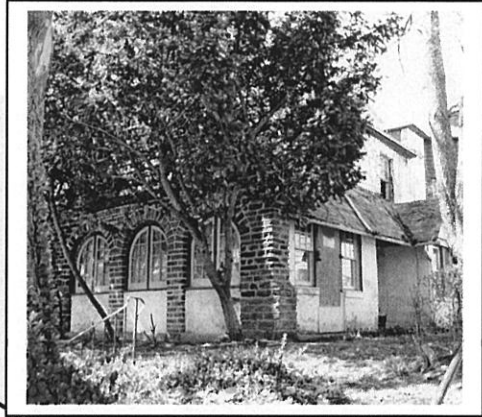
Vacant home on the 6800 block of Ogontz Avenue.
