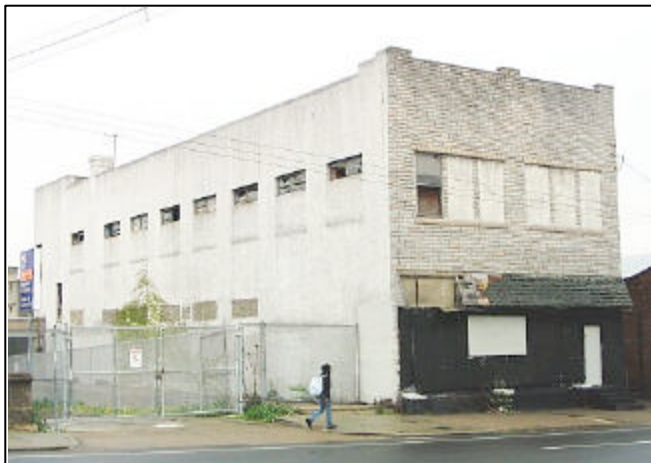
Vacant building, 1135-37 Cobbs Creek Parkway
