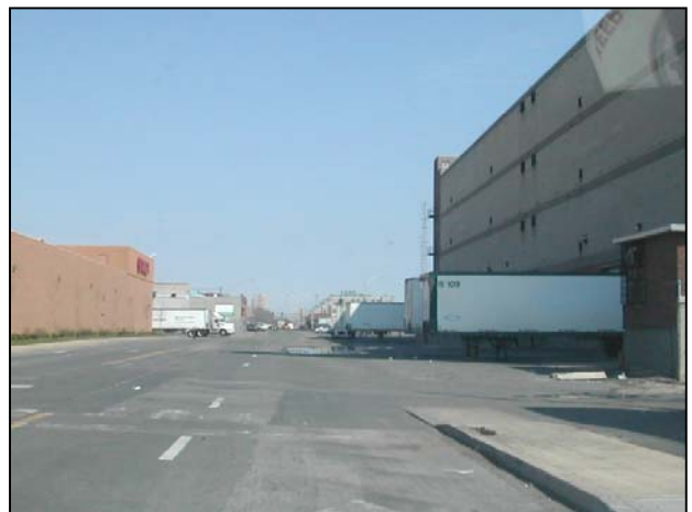
Faulty street land lot layout in the 1800 block of Swanson Street: loading dock posing a danger to vehicular traffic
