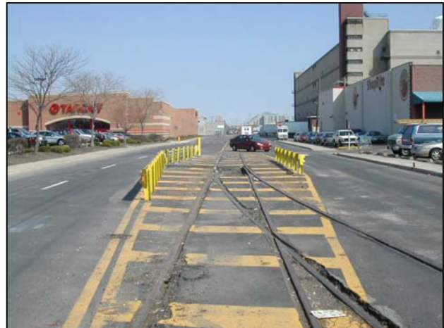
Swanson Street -- faulty street layout: Above: railroad and vehicles sharing the right-of-way. Below: confusing and dangerous traffic pattern adjacent to new retail centers located to either side of the roadway.
