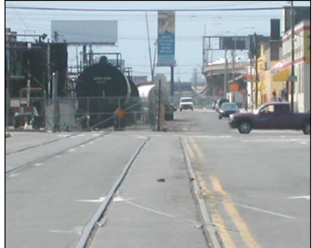
Swanson Street -- faulty street layout: Above: railroad and vehicles sharing the right-of-way. Below: confusing and dangerous traffic pattern adjacent to new retail centers located to either side of the roadway.
