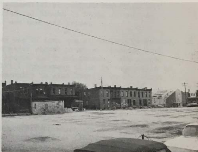
Unsafe condition of certain buildings . . . and economically underutilized land 2800 block of Lambert Street.
