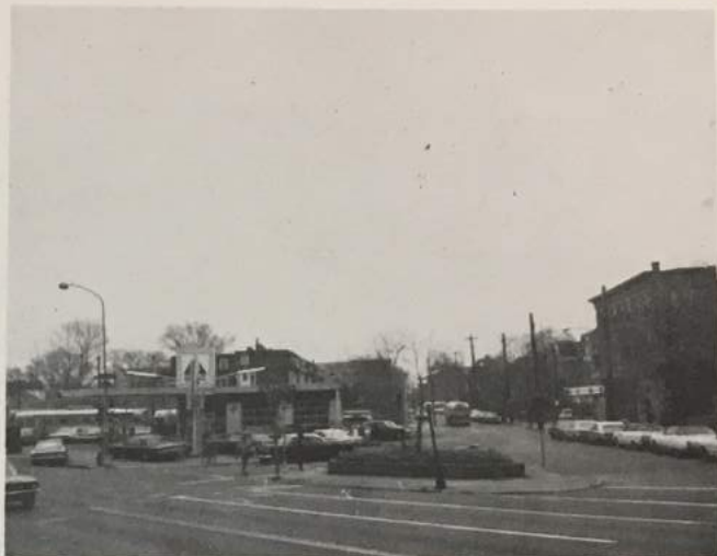
Faulty street or lot layout . . . 23rd and Venango Streets.
