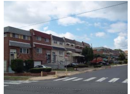
Eminent domain made possible the expansion of Temple University and the creation of Yorktown (above) in the 1960s and 1970s.
