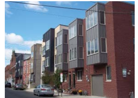
The Piazza at Schmidt's, at 2nd Street and Girard Avenue (top) is a $100 million project funded by a private developer. The project contains 430 market-rate apartments and 100,000 square feet of commercial space, including a 51,000 square foot grocery store.
